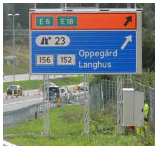
Figure 2.8 Example of a mechanically variable sign/prism sign (with outside lighting).
