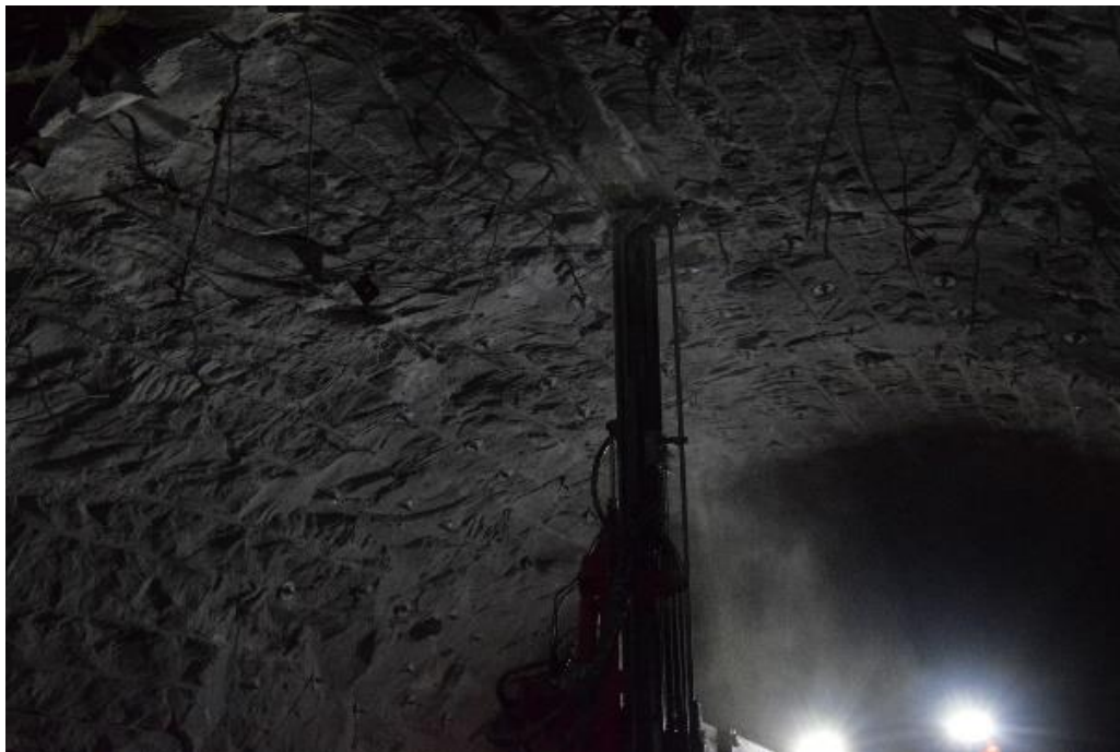
Figur 14, Boring for sikringsbolter
