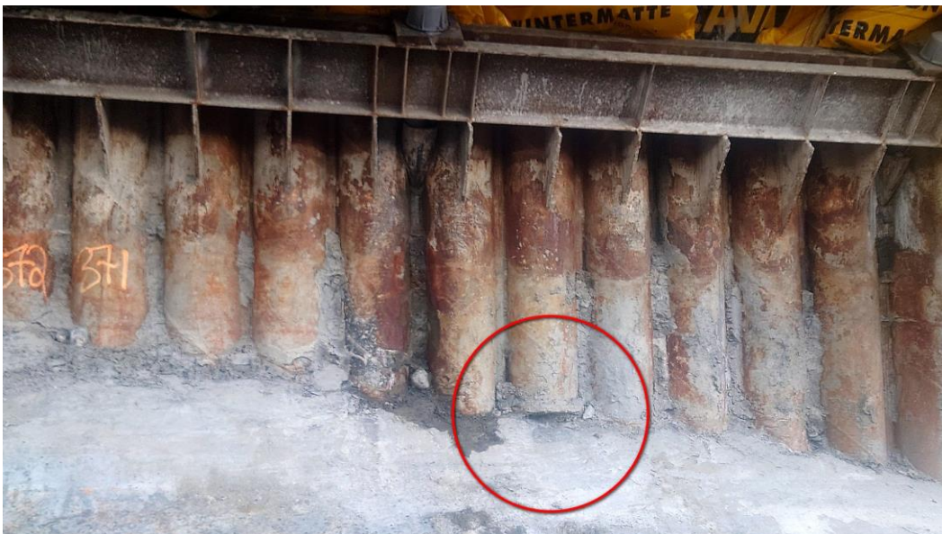
Figur 19: Rør stoppet over berg (innboret noe i bakkant)
