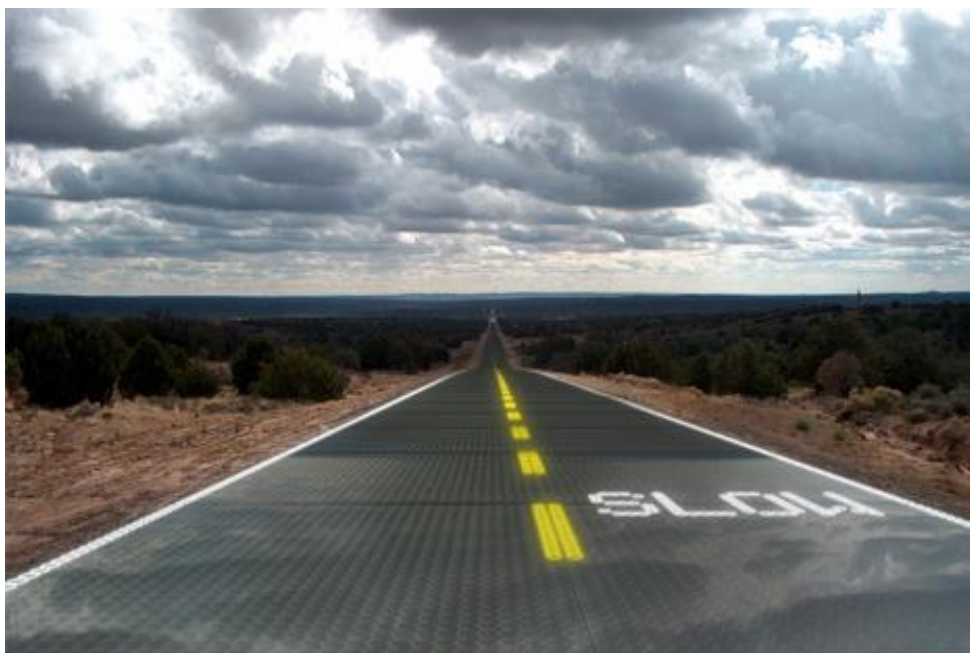
Figure 20. Dynamic road marking on smart roads.
