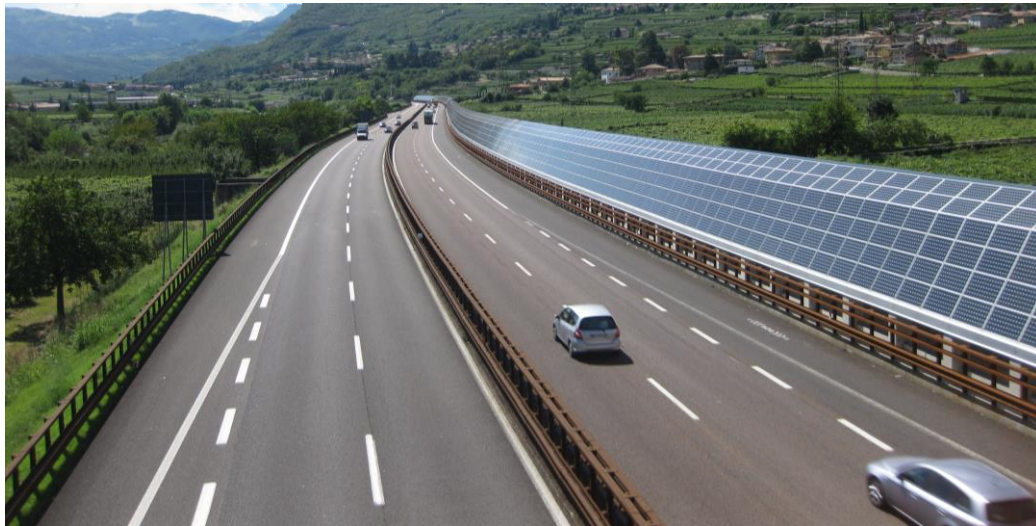
Figure 9. Solar cells installed as highway sound barriers.
