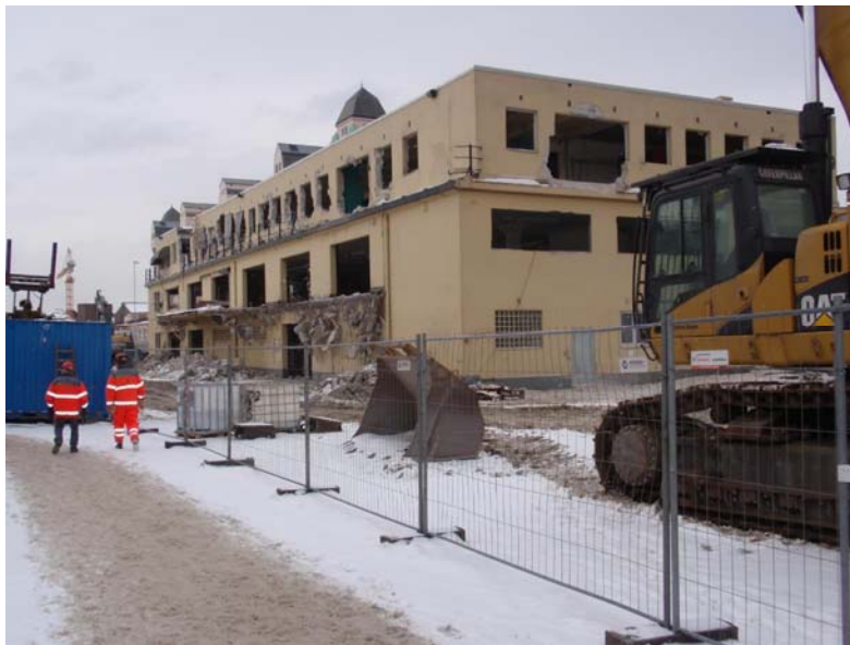
18.2.2010 – Betongramper gnages vekk
