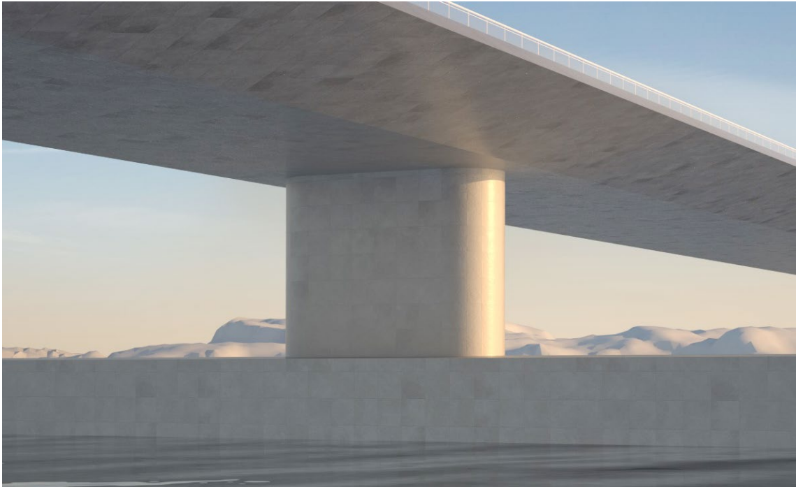
> Figure 6-2: The column given in the 0-alternativ has dimension of 4 x 8 meters.
