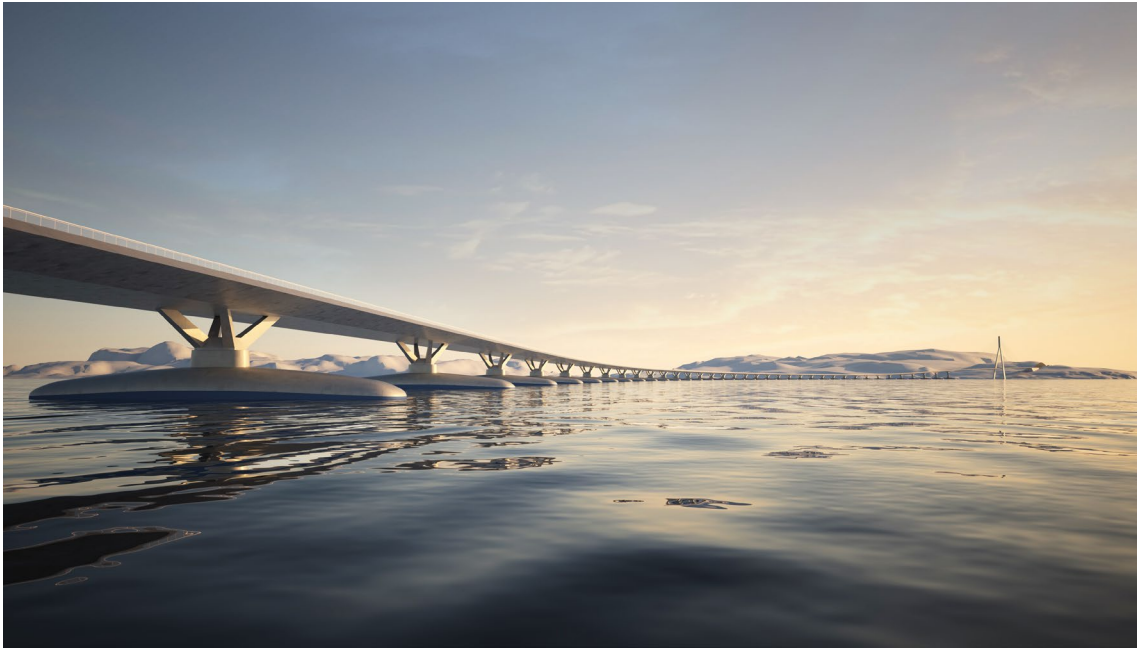
> Figure 6-9: Floating bridge with pontoon, column and rig. Seen towards the south. The pontoon close for the view
