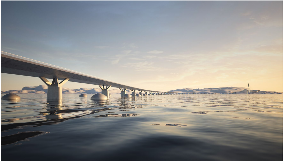
The bridge seen towards the south, submerged pontoon and steel rig column
