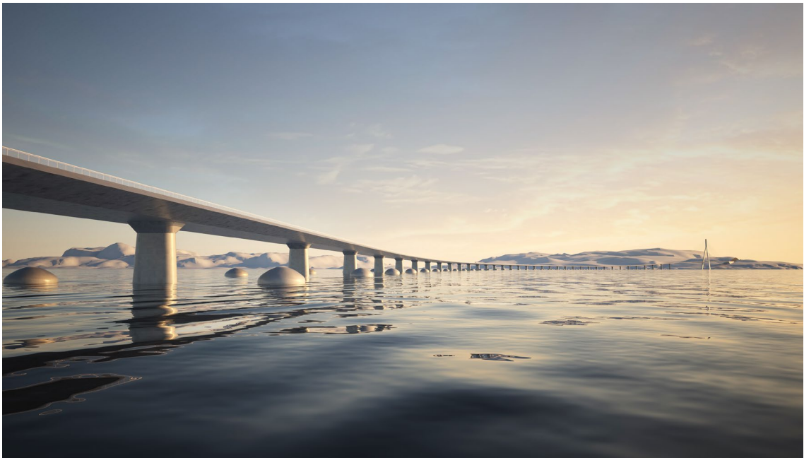
> Figure 6-10: Floating bridge with submerged pontoon, column and rig. Seen towards the south. The submerged pontoon open up for the view along the fjord
