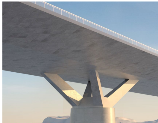
Cone-shaped column with steel rig on top
