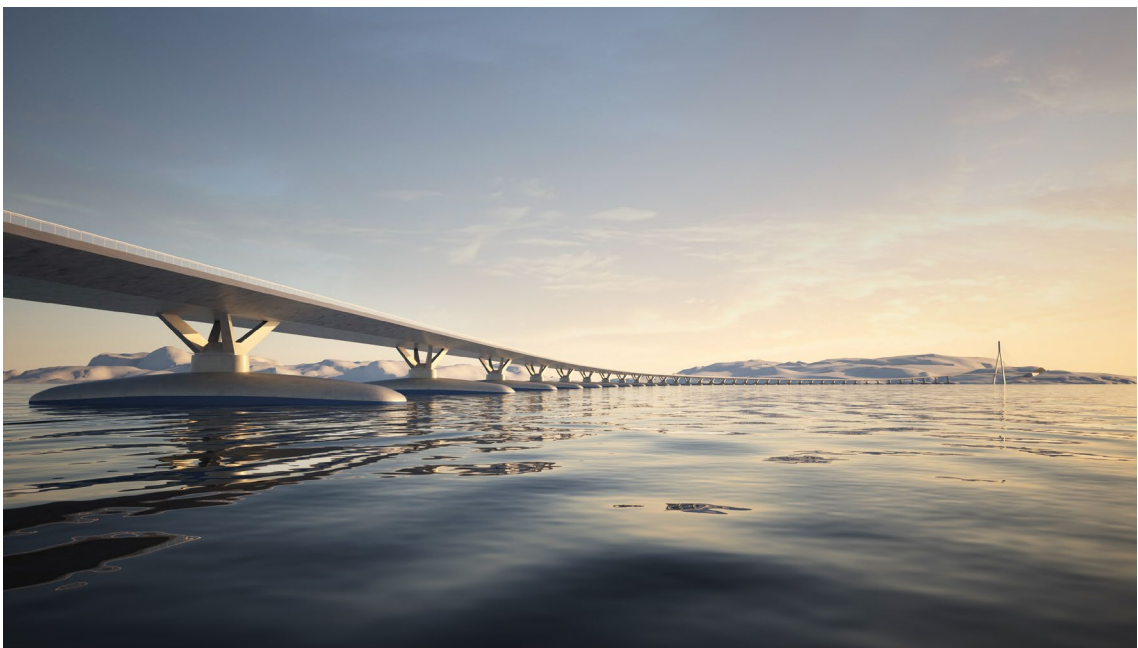
The bridge seen towards the south, floating pontoon and steel rig column
