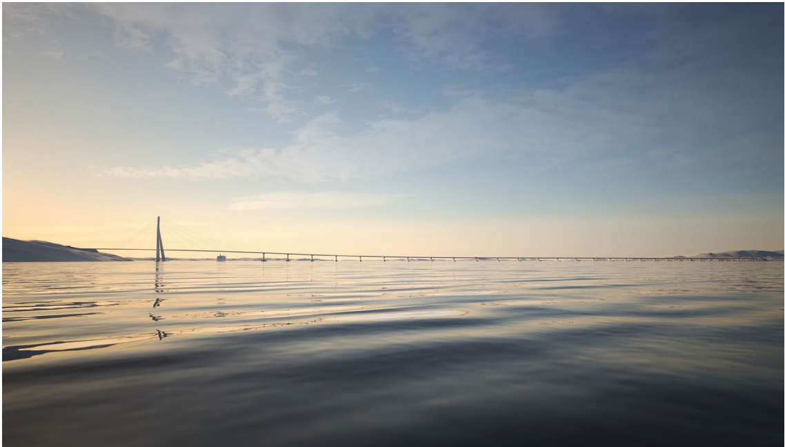
> Figure 3-3: Asymmetric cable-stayed bridge with tilted tower, seen towards the west
