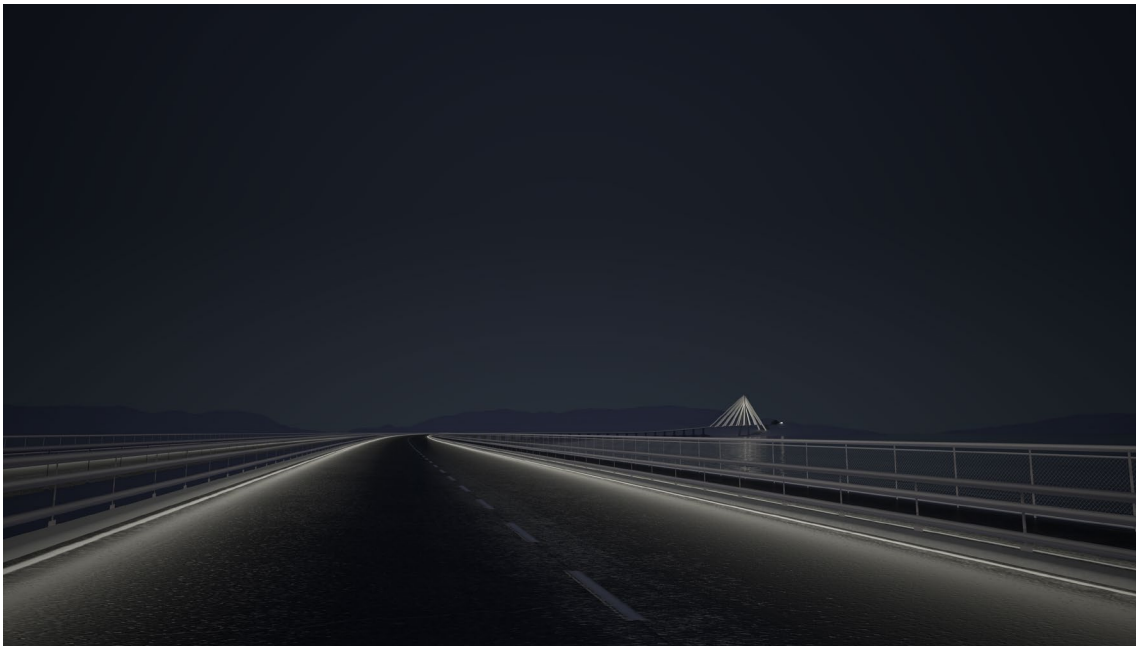
> Figure 7-1: Reduced road light from edges only. Marking the white line at night.
