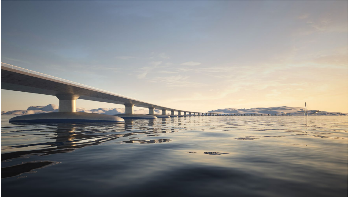
The bridge seen towards the south, floating pontoon and cone-shaped column
