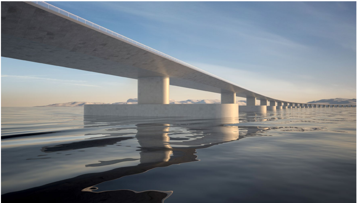
> Figure 6-3: 0-alternativ. The pontoons do not look like they are floating. They are more similar to foundations standing on the bottom of the fjord. The dimensions of the pontoon and columns can, in certain angles, create a visual wall across the fjord.
