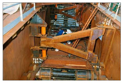
Figure 10-15 Pont de Normandie, jacking arrangement for vertical bridge positioning
