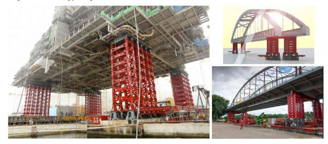
Figure 7-7: Examples of jacking towers (from ALE)
