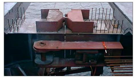
Figure 10-12 Öresund bridge, jacking system for longitudinal bridge direction
