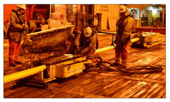
*Figure 9-7 Installation of wire grippers on wire. Used for deployment during Skarv Mooring installation (© Stefan Schlömilch)*
