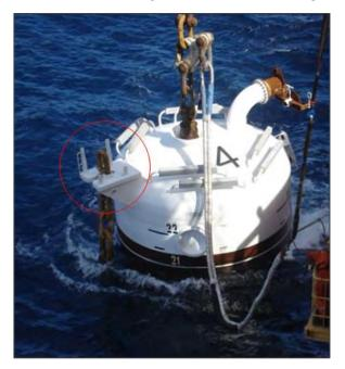
Figure 9-9 Installation of anchor with bottom chain connected at anchor hang-off table (Photo by Vicinay)
