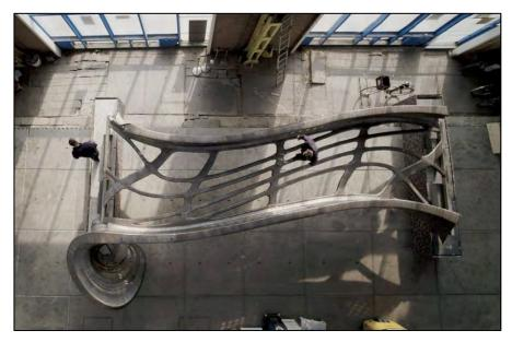
*Figure 4-28 Bridge entirely made of weld metal (3-D printed) by means of robotic welding. MX3D project, Amsterdam*
