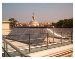
Figure 1. Installation using flat plate collectors. Foto: Arcon/ESTIF
