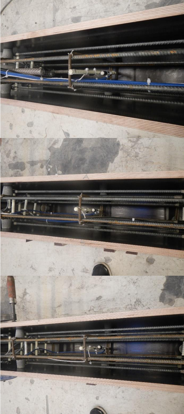
Concrete element H3 - just before casting
