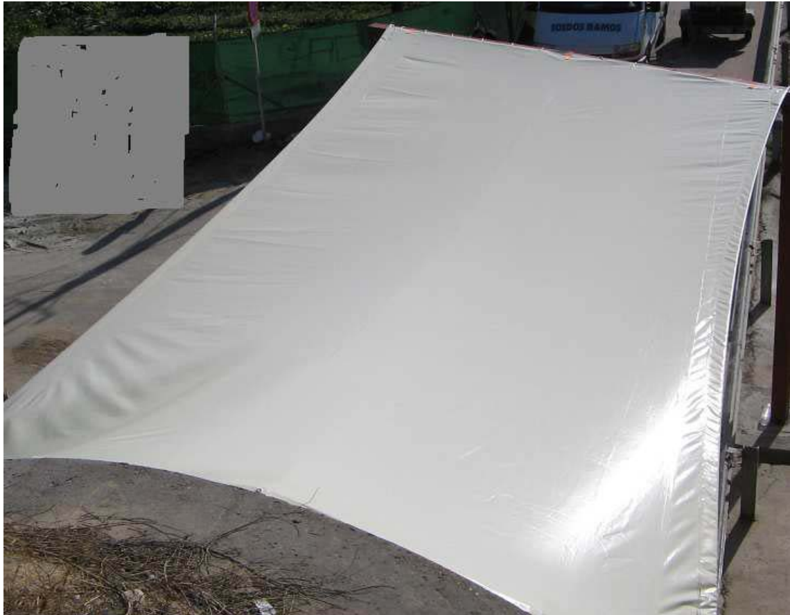
Photography 3.3. – Artificial structure to illuminate the threshold region of a road tunnel
