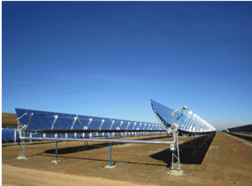
Photography 2.2.3.I. – Cylindrical parabolic collector
