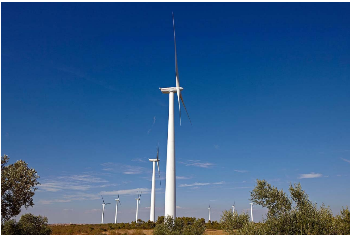
Photography 2.2.3.III. – Aero generators of 3MW power
