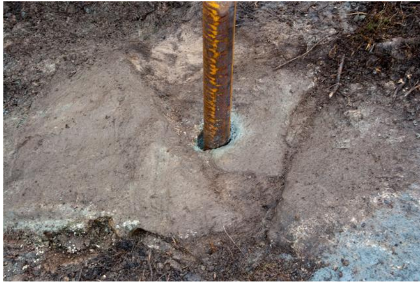
The rock with predrilled holes with the dowel driven for Shoe no. 1.
