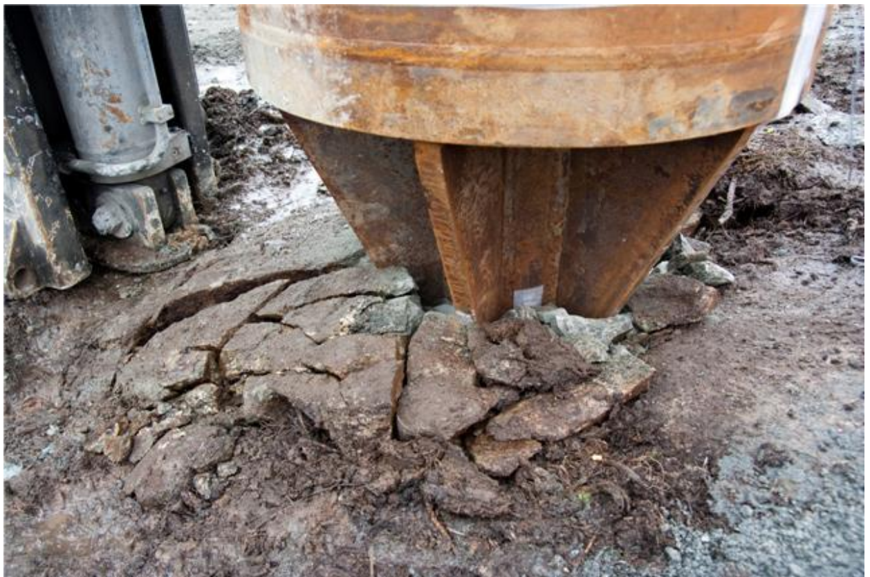
Fractured rock after the shoe had been driven down.
