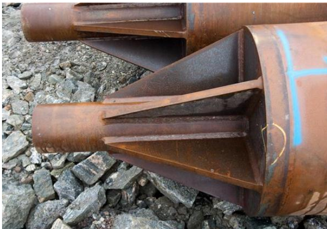
Shoe no. 1 and 2 have a base plate thickness of 80 mm
