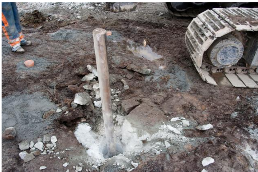
The rock with predrilled holes with the dowel driven for Shoe no. 1.
