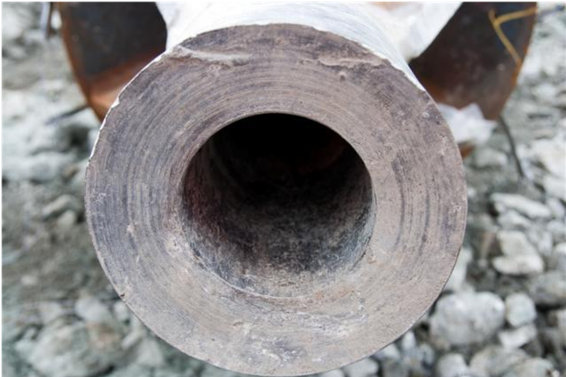
Lower edge of shoe surface after the shoe was driven.
