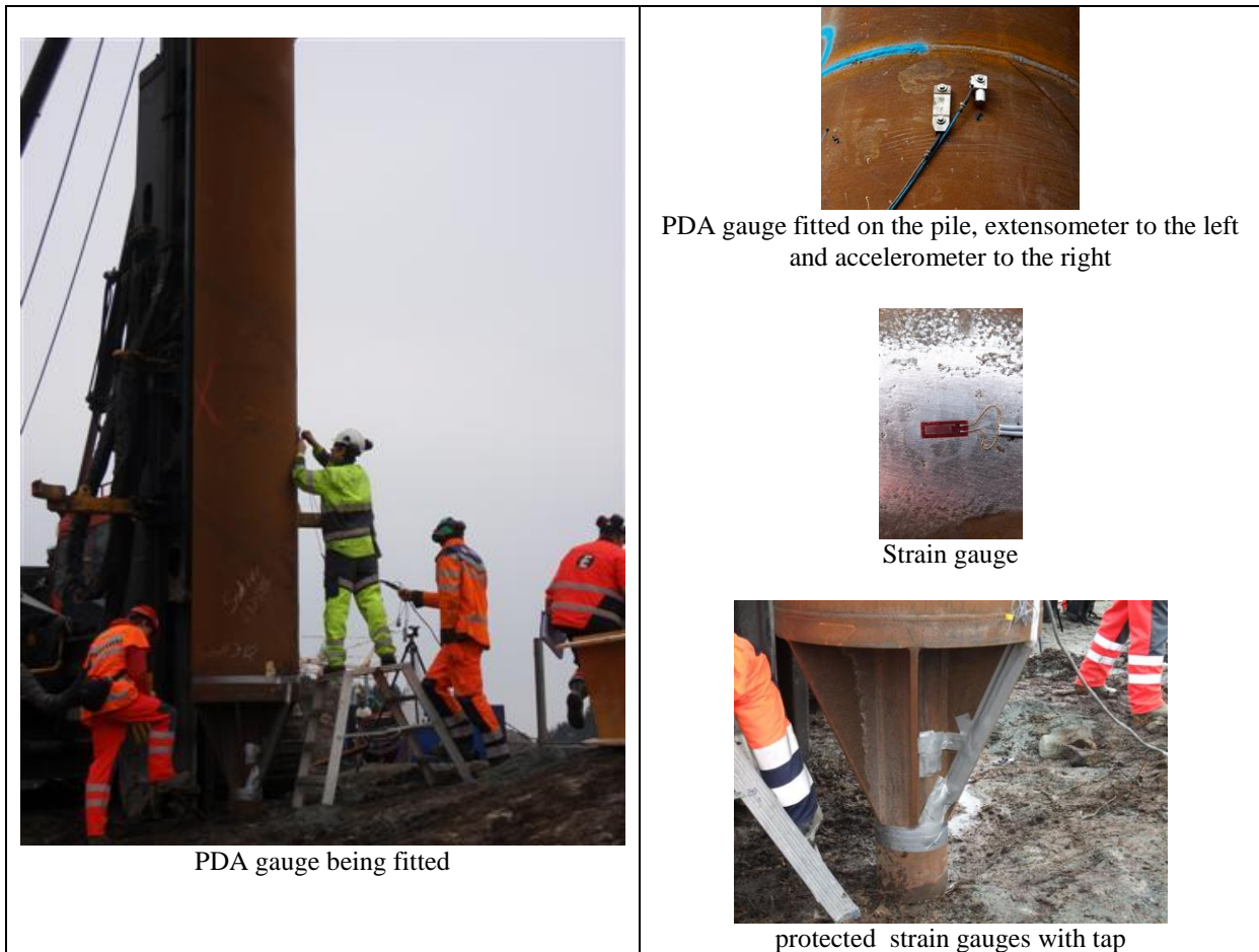
Figure 5-6: Instrumentation on the piles
