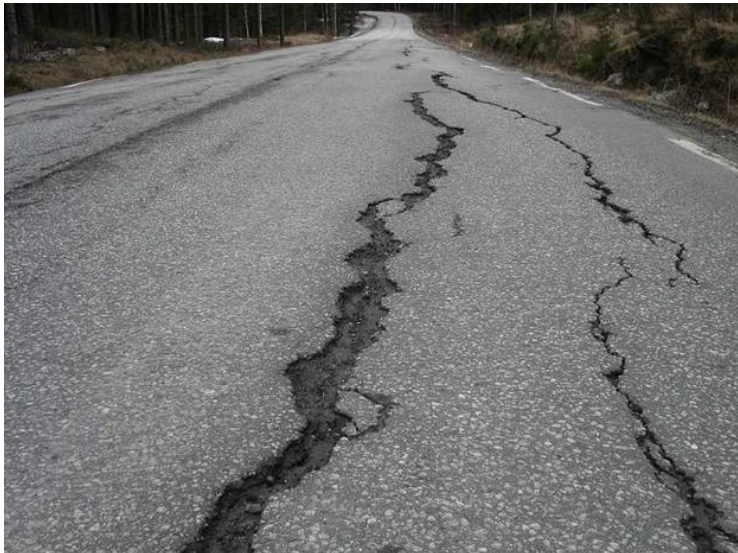
Figur 8.10 Langsgående telesprekker
