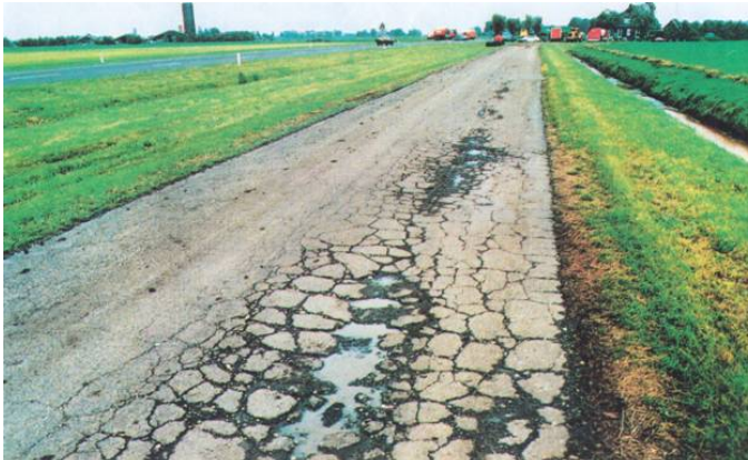
Figur 8.12 Gammelt, krakelert dekke
