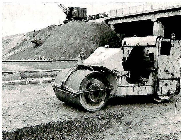
Fig. 6. Compacting lean concrete with a 1-tonne vibratory roller.
