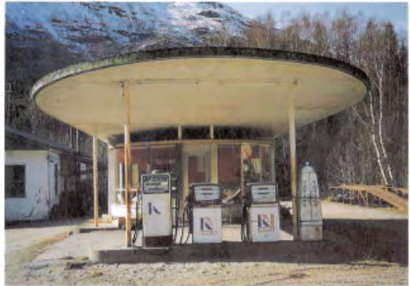
Figure 1.24 There are very few old filling stations and service stations left. This filling station from the 1950s in the Modern Movement style has recently been preserved. Luster, Sogn og Fjordane. Photograph: Birger R Lindstad, NIKU.
