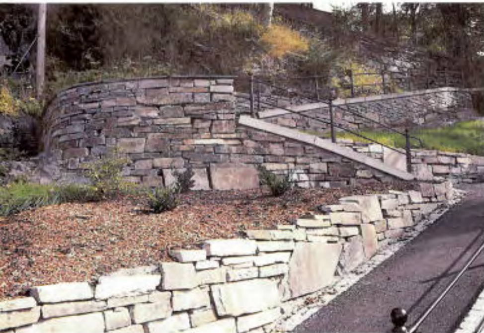
Figure 11.4 Tunnelling work for the Fløyfjells tunnel in Bergen entailed major encroachments. Exact registration was carried out beforehand. Later, the park was rebuilt using new materials which were in keeping with the original cultural environment. Photograph: Tone Høyland Stople.
