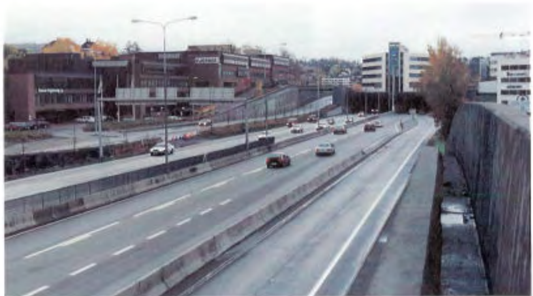
Figure 1.22 The E18 at Lysaker, Akershus. The top picture shows the road formation at the beginning of the 1960s. It was constructed to a high architectural standard, well-adapted to the surroundings. Photograph: unknown. The lower picture shows the same stretch of road in 1996. Increased traffic and other standard requirements have led to the widening and rebuilding of the road. The road construction with its neighbouring buildings now resembles architectural chaos. Photograph: Amund Vik
