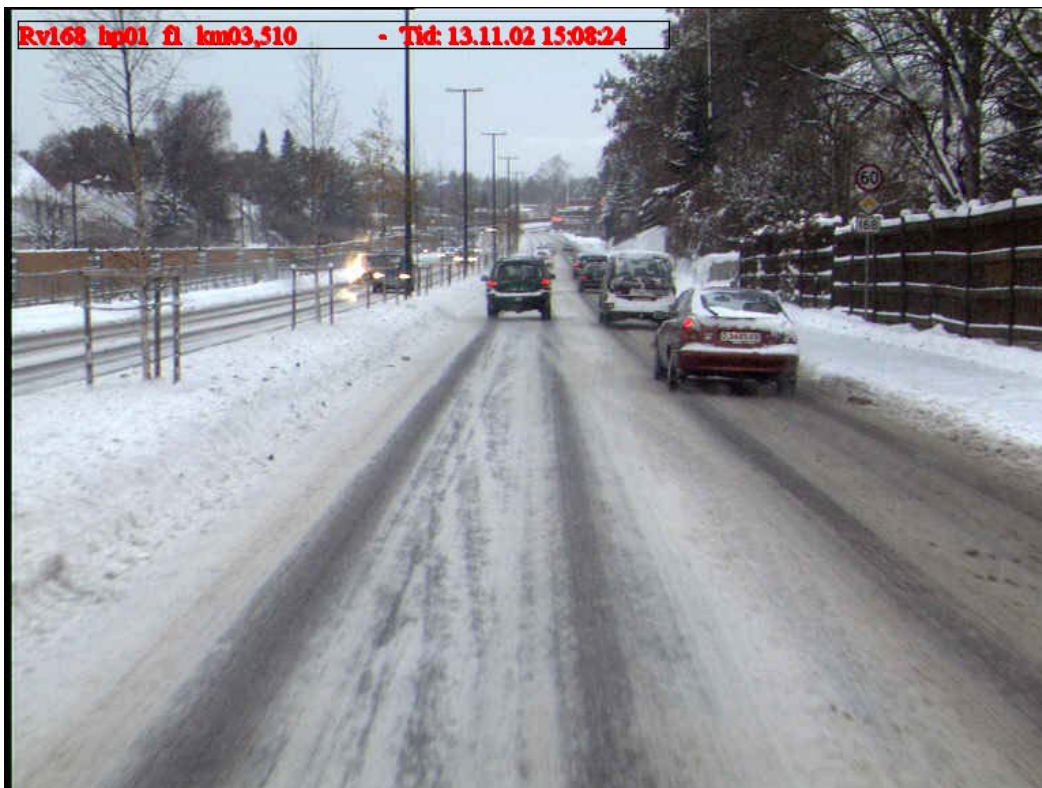
Figur VI.16: Rv 168, ny asfalt
