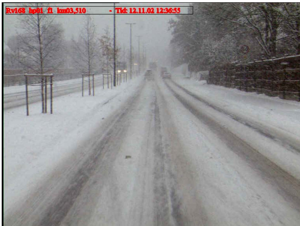
Figur VI.4: Rv 168, ny asfalt
