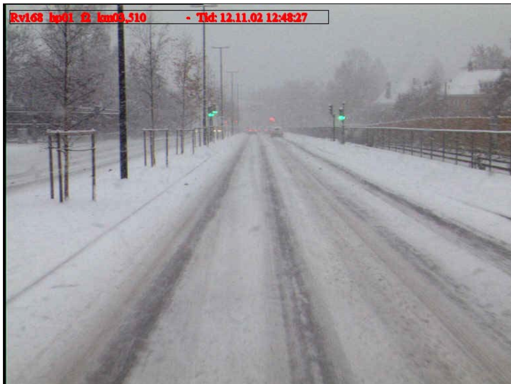
Figur VI.6: Rv 168, ny asfalt
