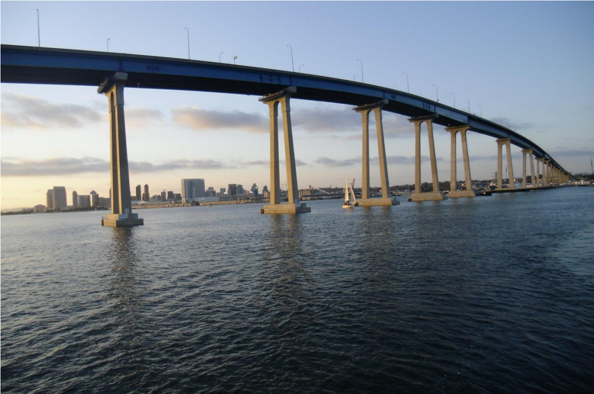
San Diego Coronado Bay Bridge
