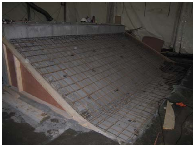
Ferdig armert felt i streetanlegg.
