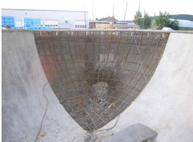
Ferdig armert felt i bowlanlegg.
