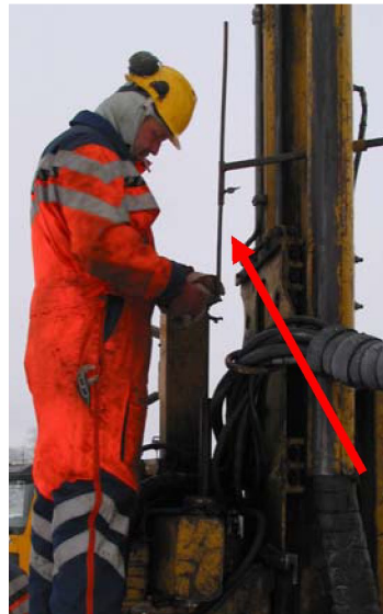
Figure 18 "gallows" for fixation of inner rod
