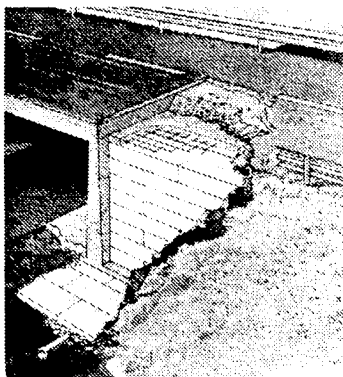
Figure 2.4 Reduced lateral pressure. E 18 Sem, Norway.
