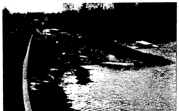
b) Water fluctuation. Rv 159 Flom bridge, Norway.
