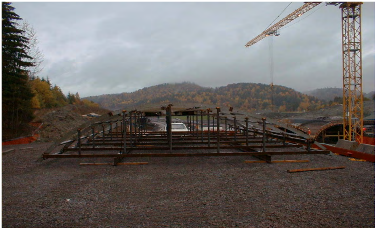
Figur 5. Monteringsmal for hvelvarmeringen
