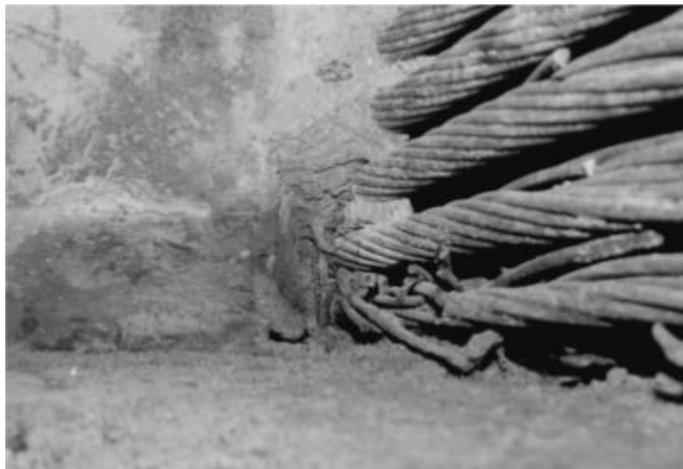
**ID-28.1.** Corrosion of external tendons that had been encased in concrete (Tilly, 2002).
