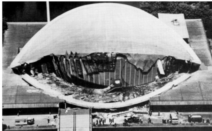
**ID-19.5.** View from the South on the collapsed roof overhang in 1980 (Helmerich and Zunkel, 2014).
