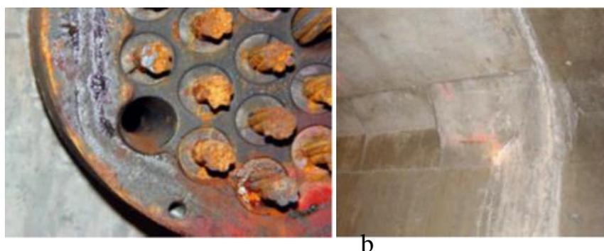
**Figure 3.1.10.** San Francisco – Oakland Bay Bridge (ID-14): a) close-up view of an anchorage head showing signs of corrosion from water collected at the anchorage; b) view of a crack at an anchor block showing efflorescence (Reis, 2007).
