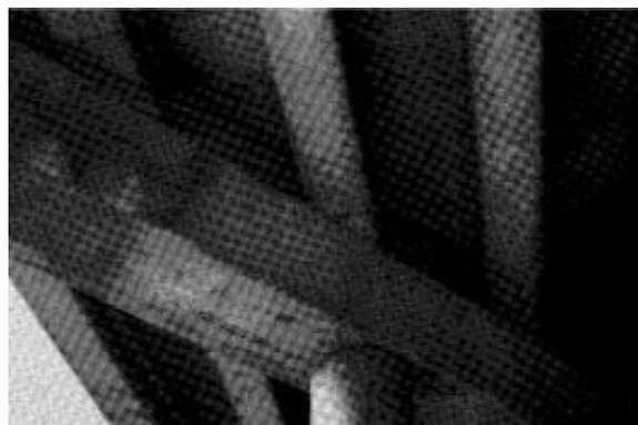
**Figure 3.1.24.** Harlem Avenue overpass, USA (ID-32). Corrosion of the bottom of the girder. (Gustafarro et al, 1983).
