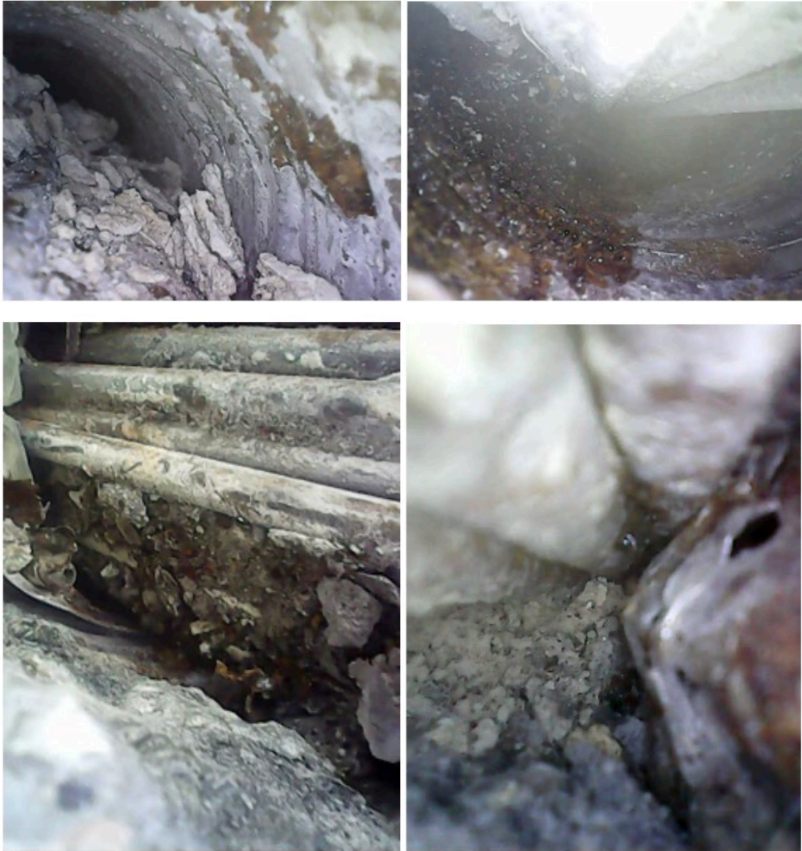
Figure E.4: Images taken from inspection site 1. Corresponds to image E2-1 to E2-4 in Appendix F, respectively
