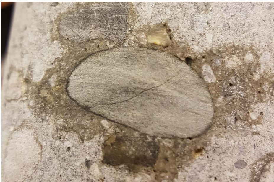
Figure 5-29 closeup of reactive aggregate in core M6.
