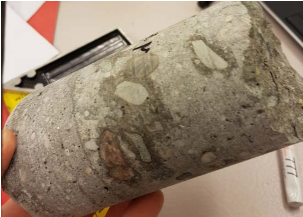
Figure 5-30 M6 showing several potential reactive aggregates, with surrounding moisture
