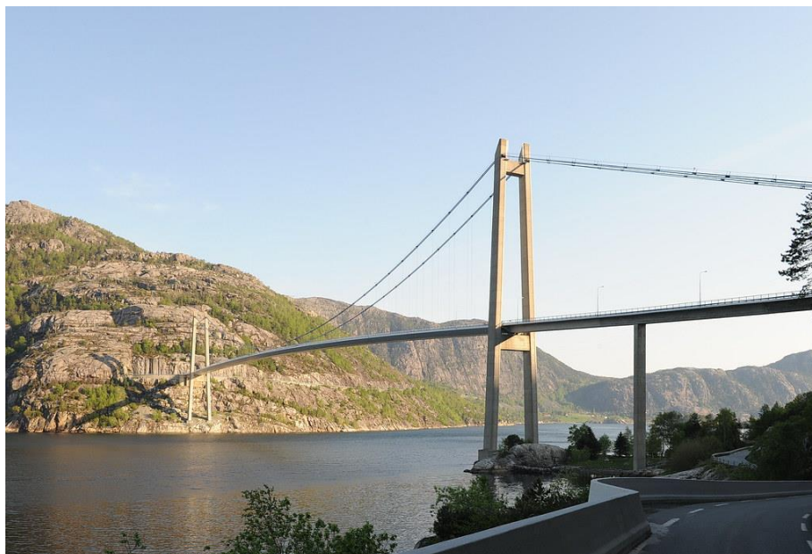
Figure 1 View of the Lysefjord bridge from the southwest, from [1]
