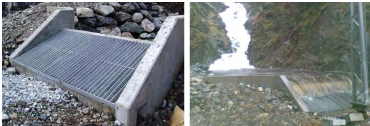
Figure 3.6: Self cleaning grids in Langhelle. On the right is the self cleaning grid during a flooding (Photo: John Endre Fossmark) and the left when there is normal flow (Photo: Jeanette Gundersen).
