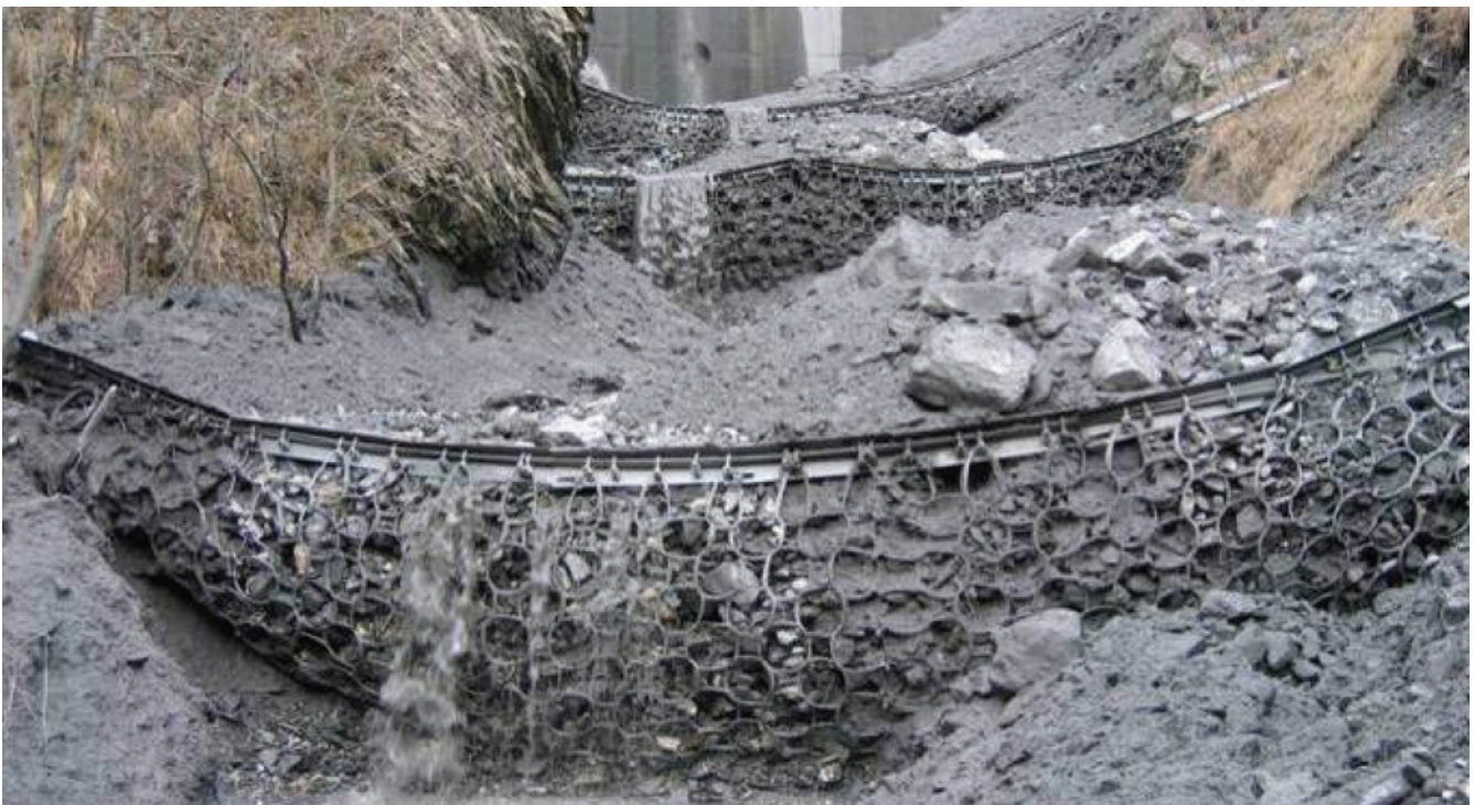
Figure 2.9: A multi-level flexible barriers in the Merdenson torrent in Switzerland after stopping a debris flow (Volkwein et al., 2011).
