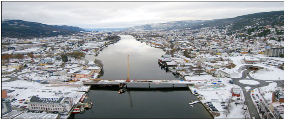
Figure 5. 1 View of øvre sund bridge prject, Drammen.
