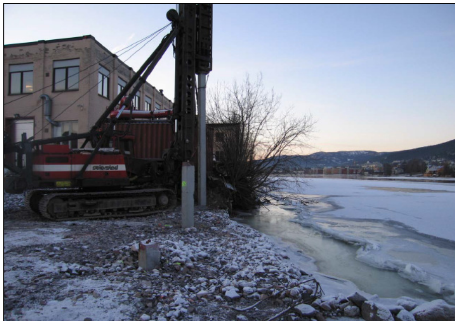
Figure 6. 3 Piling in progress at Grønland side. (Photo : Tefera T.)
