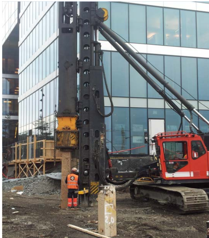
Figure 5.1 Concrete pile driving in the city of Oslo (after Ermias)
