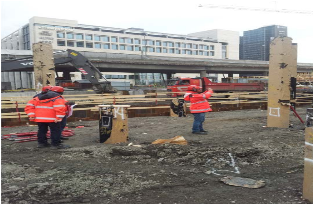
Figure 2.4 Concrete piles used as foundation material (after Ermias)
