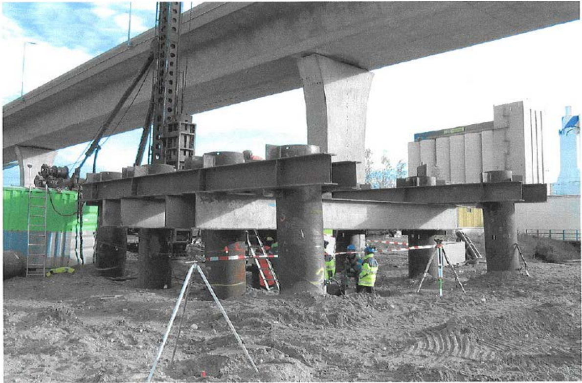
Figure 6.6 Static load test at axis 25 (after Grete Trevdt)
