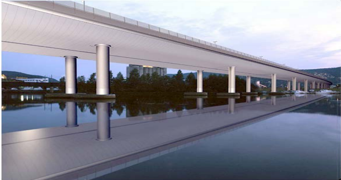
Figure 6.4 The old and the new bridge side by side after the pier of the old bridge upgraded to a circular cross section (after Grete Trevdt)
