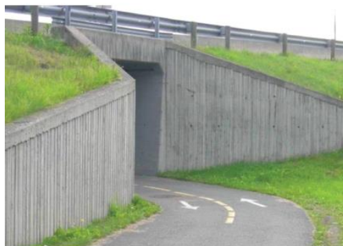
Figur 9: Planskilt kryssing via undergang (8).
