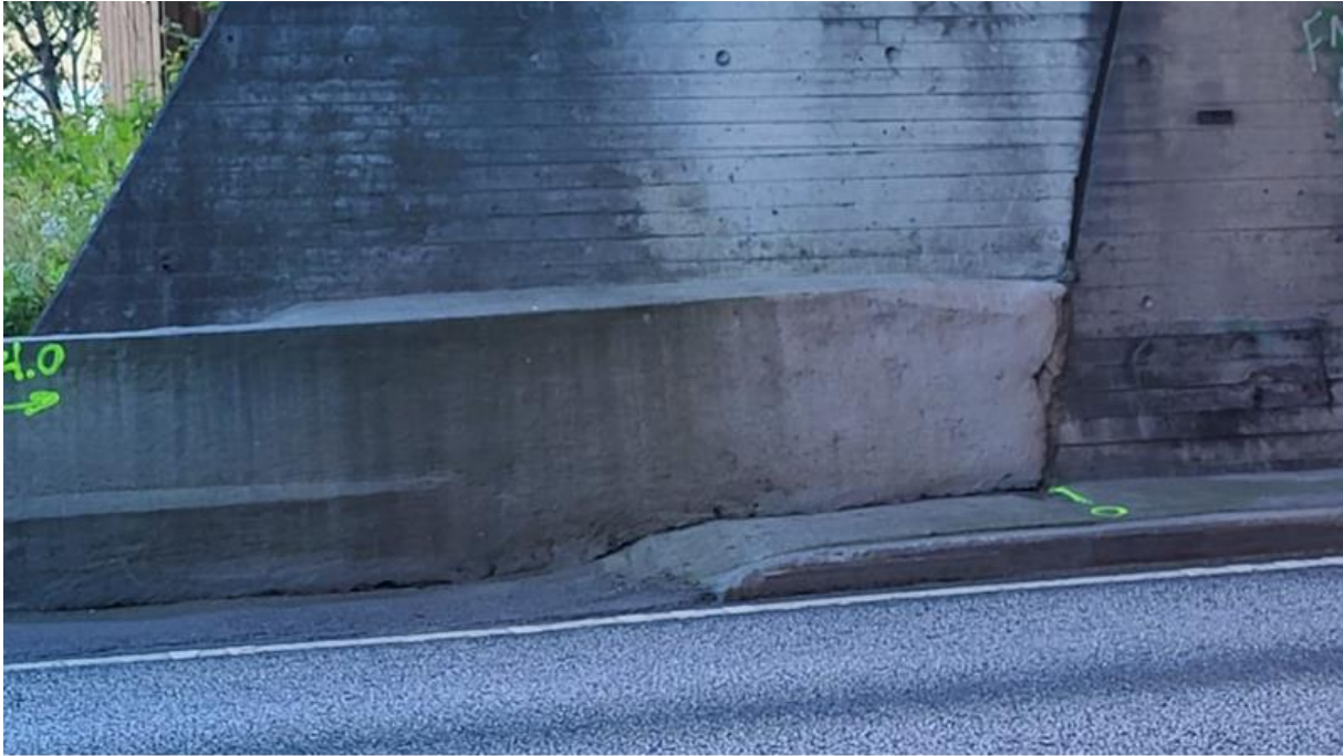
Figur 2 Measurement of fasit outside of the tunnel
