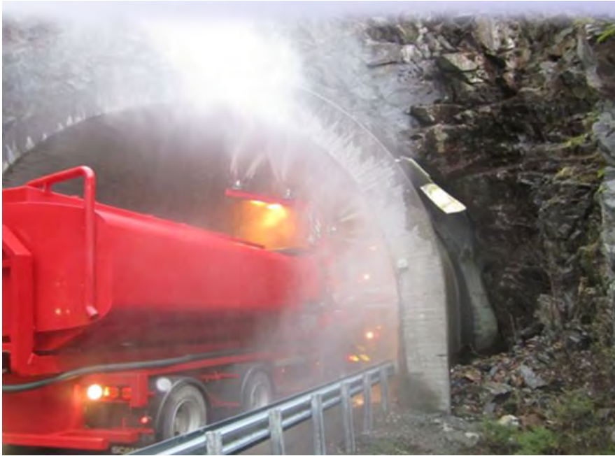
Figur 9-47 Tunnelvask (Foto: Veimas)
