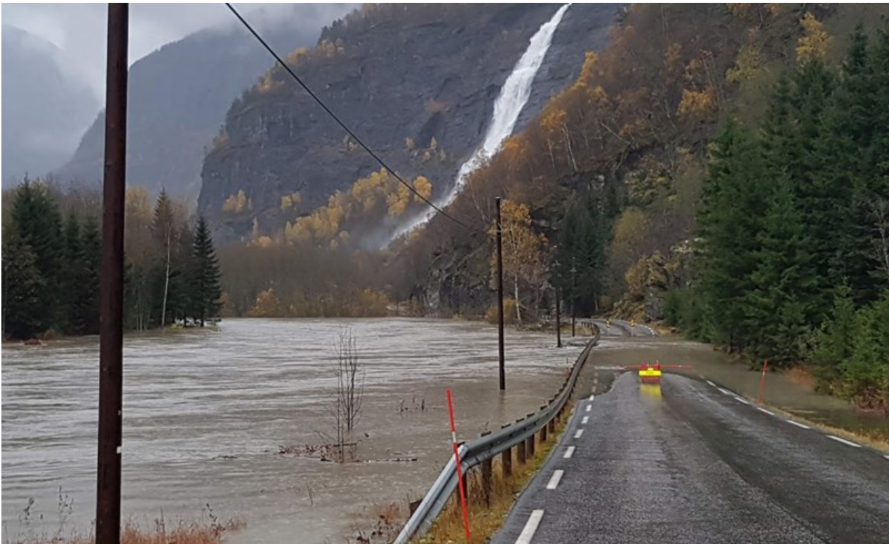
Figure 1 – National road 55 flooded from heavy rain, in October 2018, in Skjolden, Sogn og Fjordane. Photo Mari Vold, NVE.
