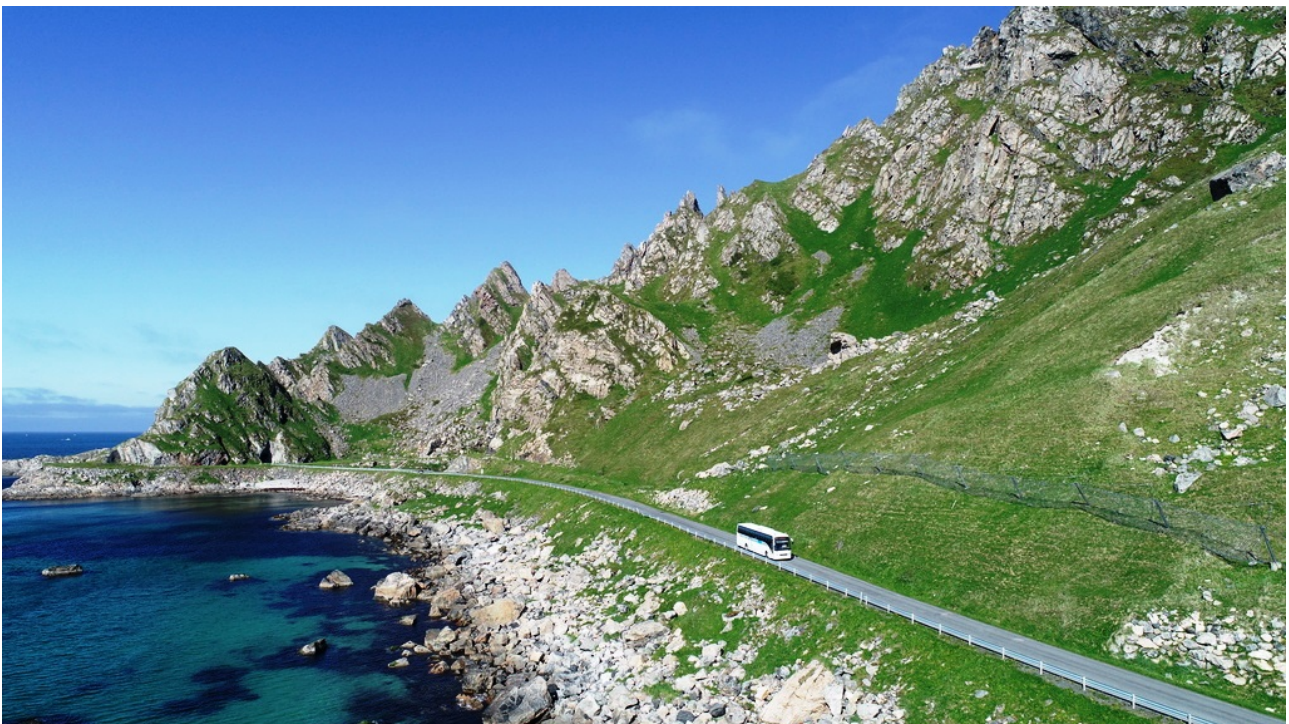
Figure 3 – Andøya island, Nordland, Norway, county road 976, with protection fences for rock fall. Photo: Tomas Rolland, NPRA
