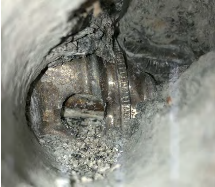
Photo no 6.4.1: Tendon duct 1SC with confirmed grouting
