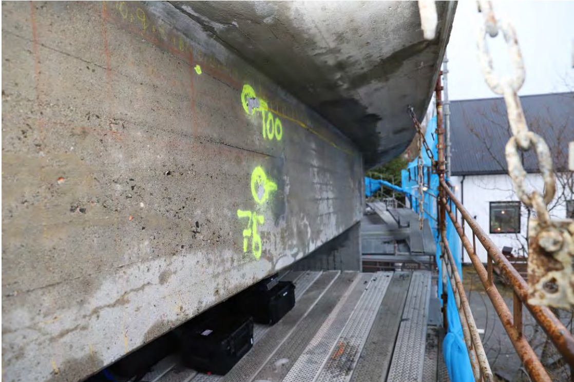
Photo 4.1: Two different visual inspection areas in girder.
