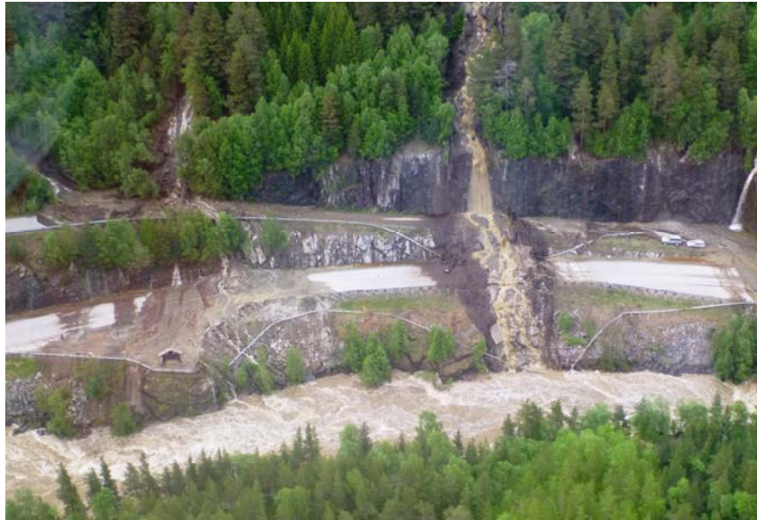
Fig. 3. Debris flow, such as over E6 in Rosten, Norway, may occur more often in a wetter climate (foto: Niklas Eriksson, NPRA)
