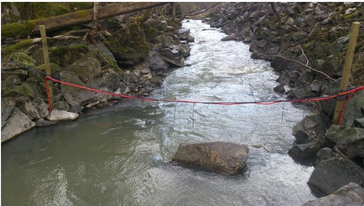
Figure 6: PTT antenna 2, mounted on the downstream end of station 4
