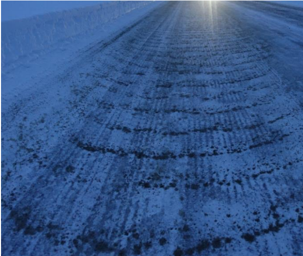
Figur 23: Fastsand Epoke flystripe (med 0/4 mm Lora).
