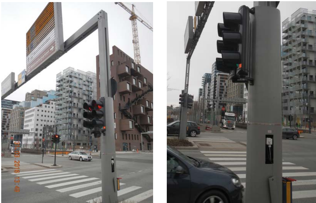
Figur 9-11 Betjeningsbryter for skiltportal i portalbeinet
