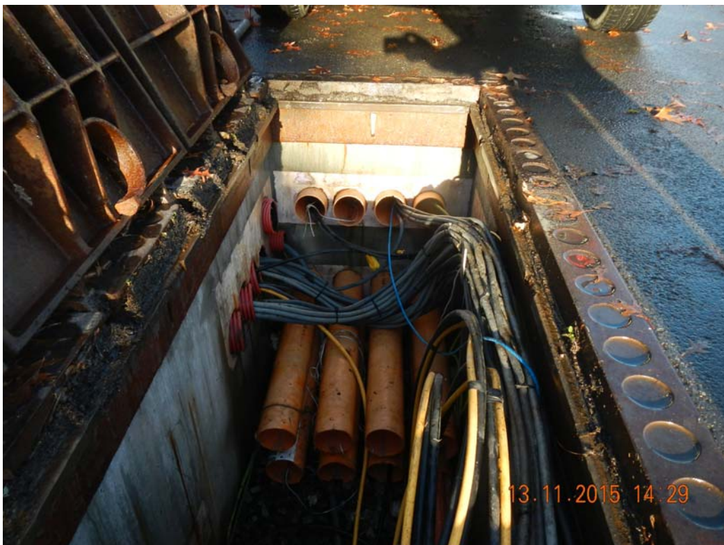
Figur 9-3 Ferdig montert trippelkum for stamrørtraseen
