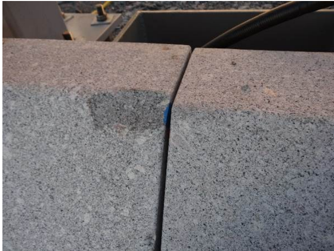
Figur 5-22 Kantsteinsfuge
