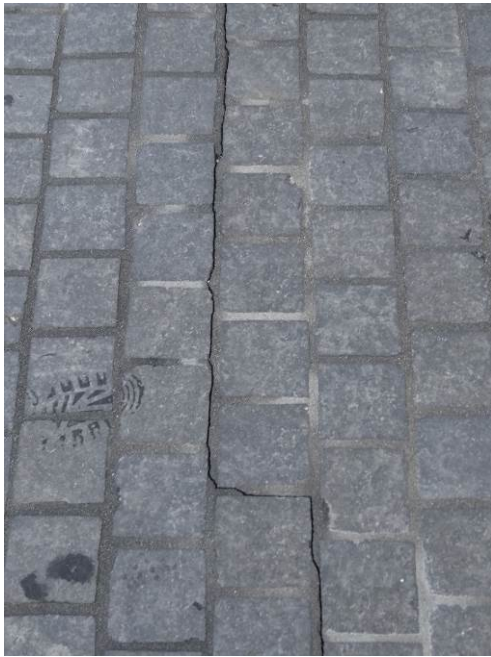
Figur 5-24 Spenningsriss i bundne gatesteinsdekke
