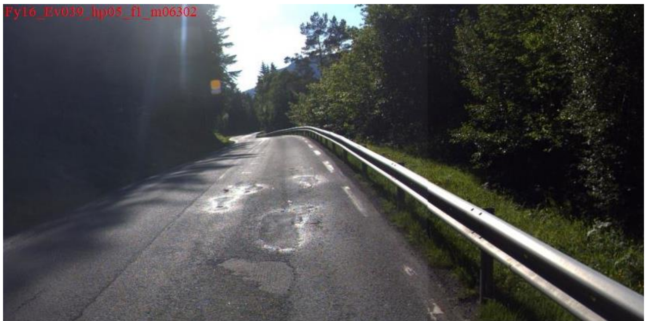
Figur 2. Ev. 39, Hp05, m 6302_13.6.16. Agb11 WAM i felt 1. Slaghull har blitt lappet.
