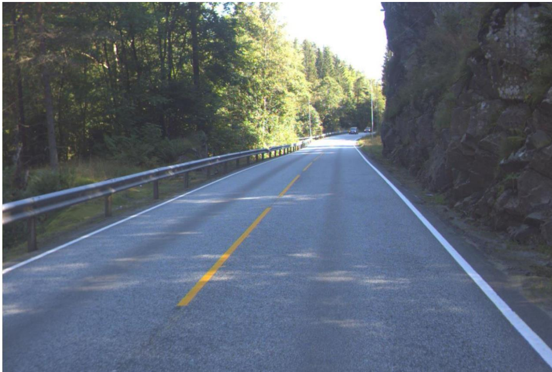
Figur 7. Rv 9, hp04, m 2114_17.8.16. Ab16 Green Asphalt i felt 2.
