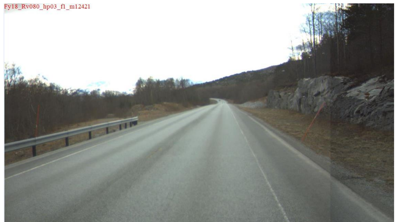
Figur 16. Rv. 80, hp03/km 12,417_26.4.16. Ab16 Cecabase i felt 1.
