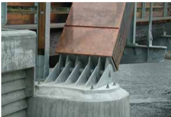
Figur 6-29: Overgurten får øket bredde mot kemperleddet for å gi sideveis innspenning Figure 6-29: Increased width of upper chord towards the impost hinge in order to establish lateral restraint
