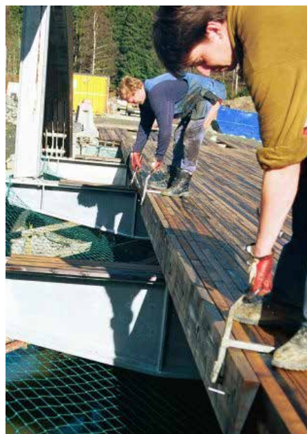
Figur 11-5: Montasje av lamellene i et tverrspent dekke Figure 11-5: Assembly of the lamellas of a stress laminated deck
