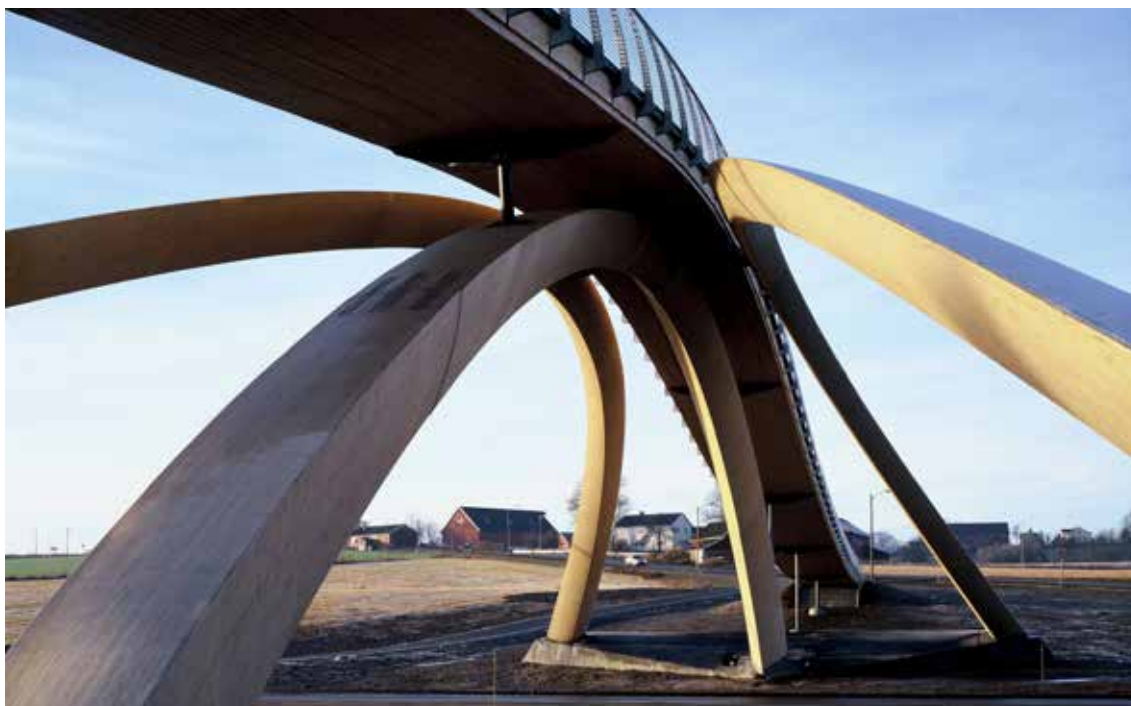
Figur 11-2: Buene til Leonardo da Vinci bru med sine dobbeltkrumme flater Figure 11-2: The arches of Leonardo da Vinci Bridge with their doubly curved surfaces
