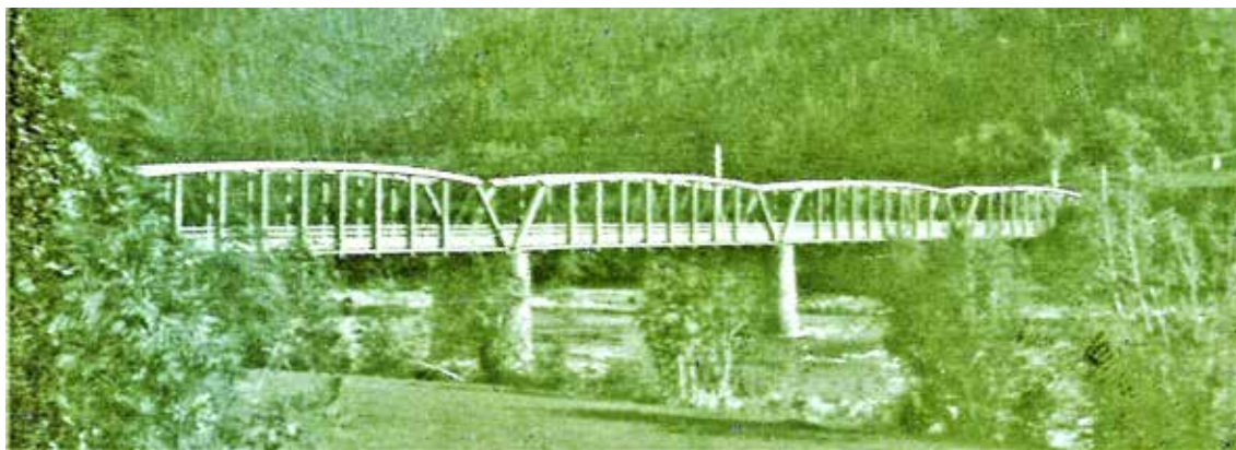
Figur 1-10: Hegra bru over Stjørdalselva Figure 1-10: Hegra Bridge over the Stjørdal River
