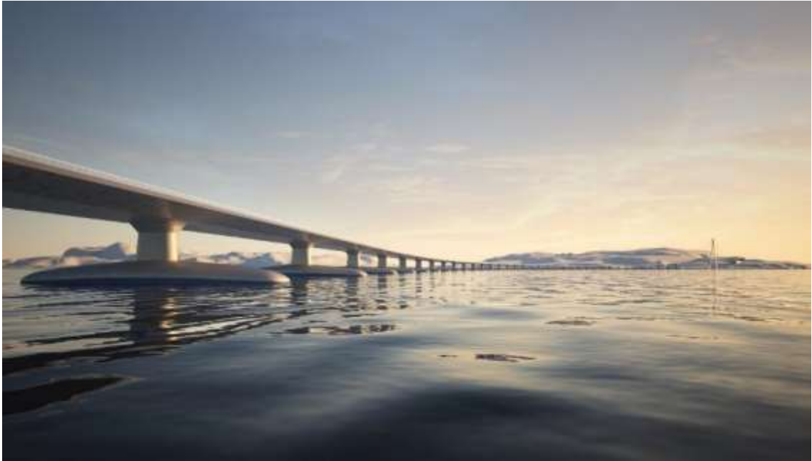
The bridge seen towards the south, option 2
