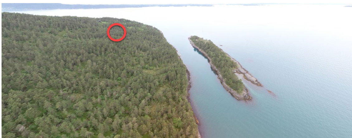
> Figure 3-11: Aerial photo of Reksteren from east, Svarvhelleholmen island to the right. The red circle indicates the abutment localization.
