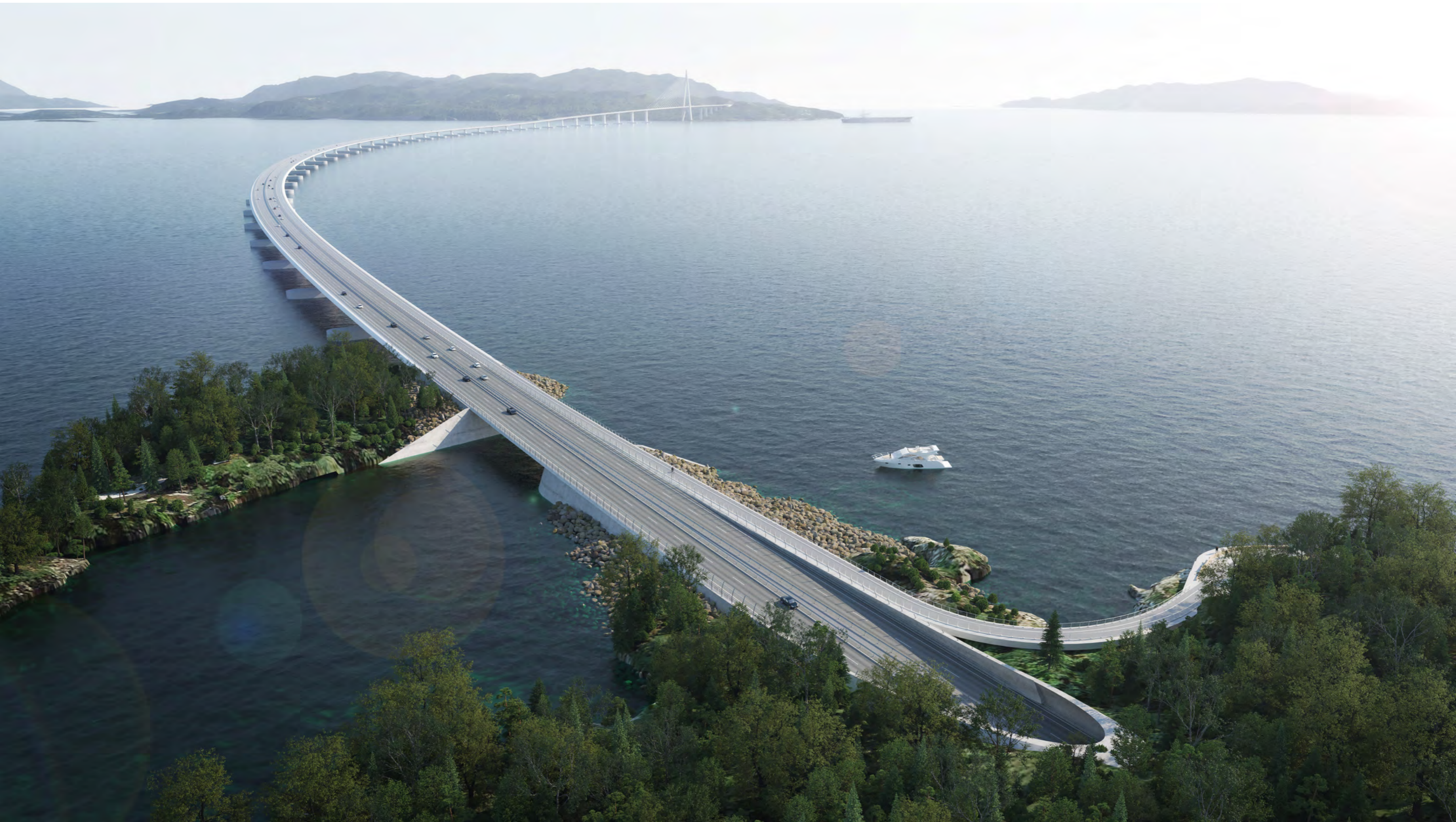
LANDING NORTH - CULVERT, TUNNEL PORTAL, VIEWING PLATFORM
