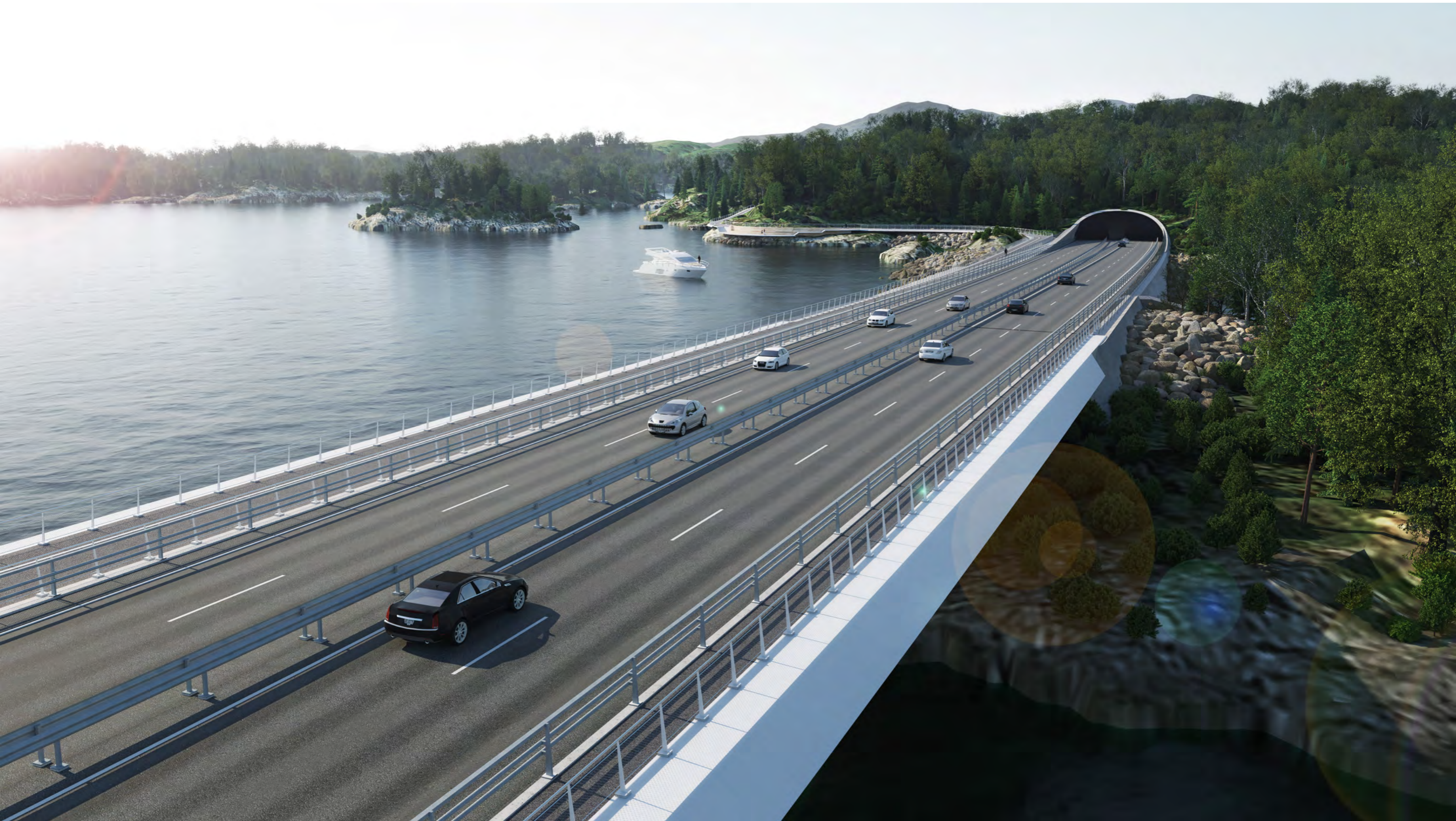
LANDING NORTH - TUNNEL PORTAL, VIEWING PLATFORM
