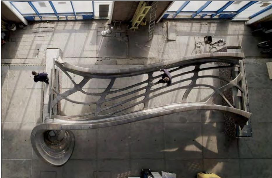
Figure 16-4 Bridge entirely made of weld metal (3-D printed) by means of robotic welding. MX3D project, Amsterdam
