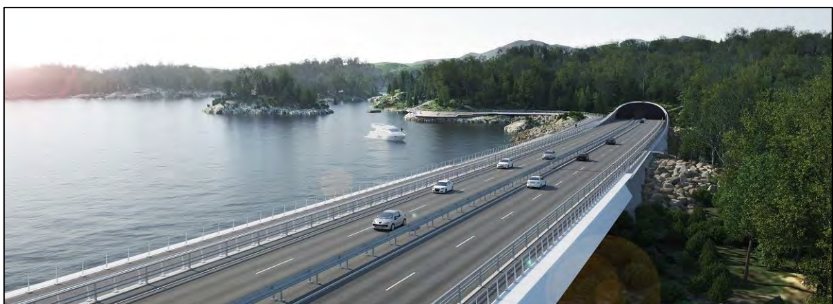
Figure 7-12 Illustration of the northern abutment and the tunnel entrance
