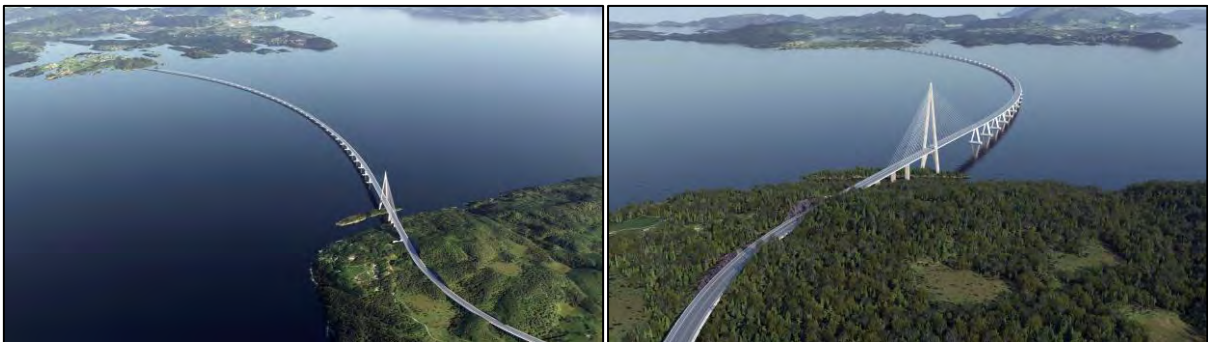
Figure 5-1 K12 - C-shaped bridge
