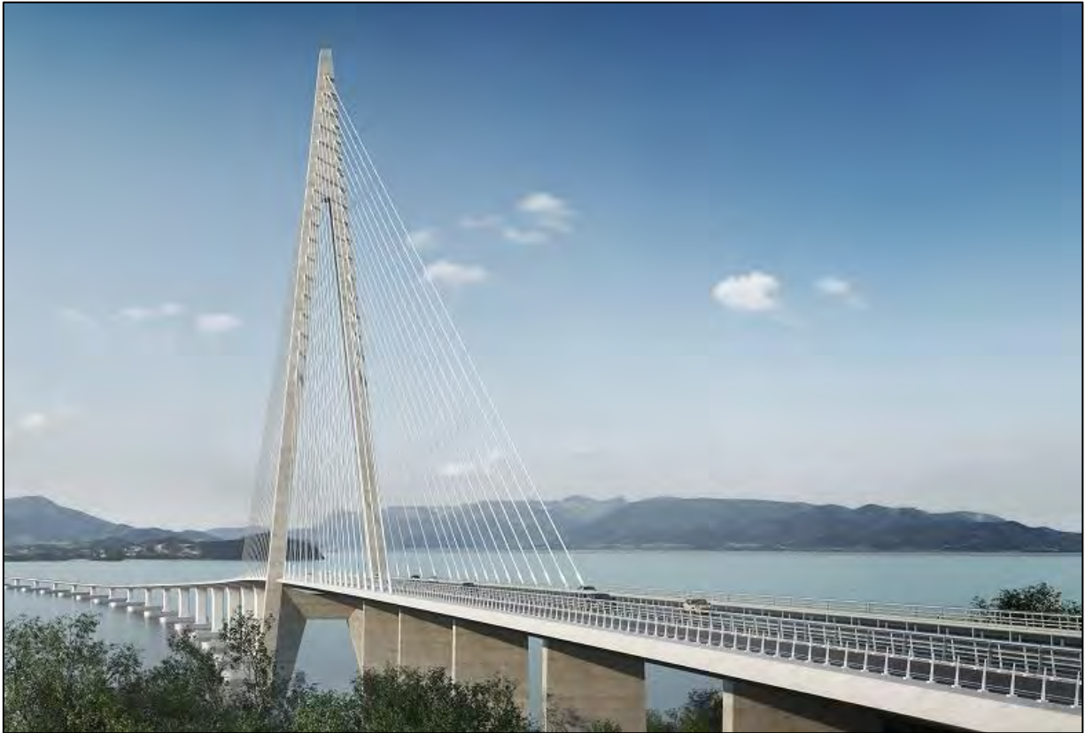
Figure 7-9 Cable stayed bridge with the tower forming a light house landmark
