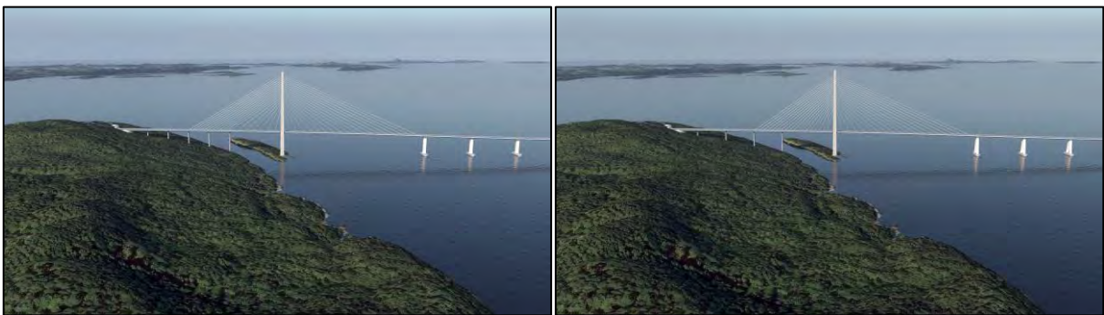
Figure 5-2 “Basecase” stay cable and back span arrangement and “optional” arrangement
