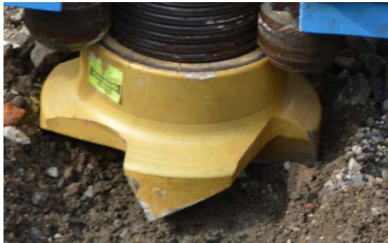
Figure 5-16. Carbide cross cut Ø340 mm, Titan 196/130, 3 m long, Coupling nut Ø254 x 600 mm.
