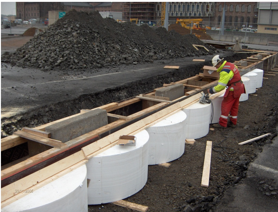
Figur 13: Mal for borerør
