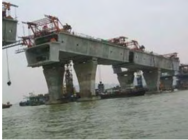
Fig. 5 Cantilever Erection of the Girder
