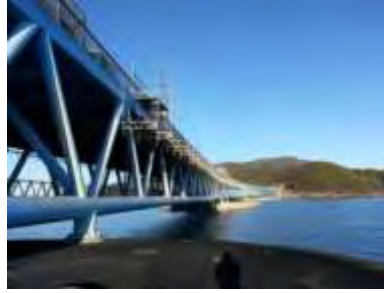
Figure 15: The Bergsøysund Bridge
