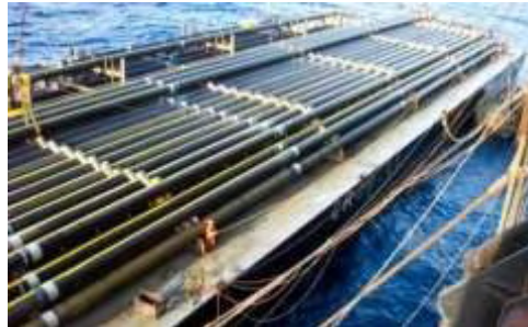
Figure 14 Tether main Body Segments Prior Installation
