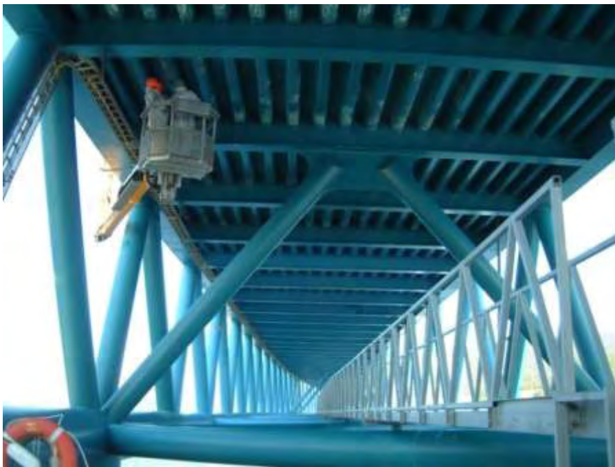
Photo no. 5 Maintenance work in progress
