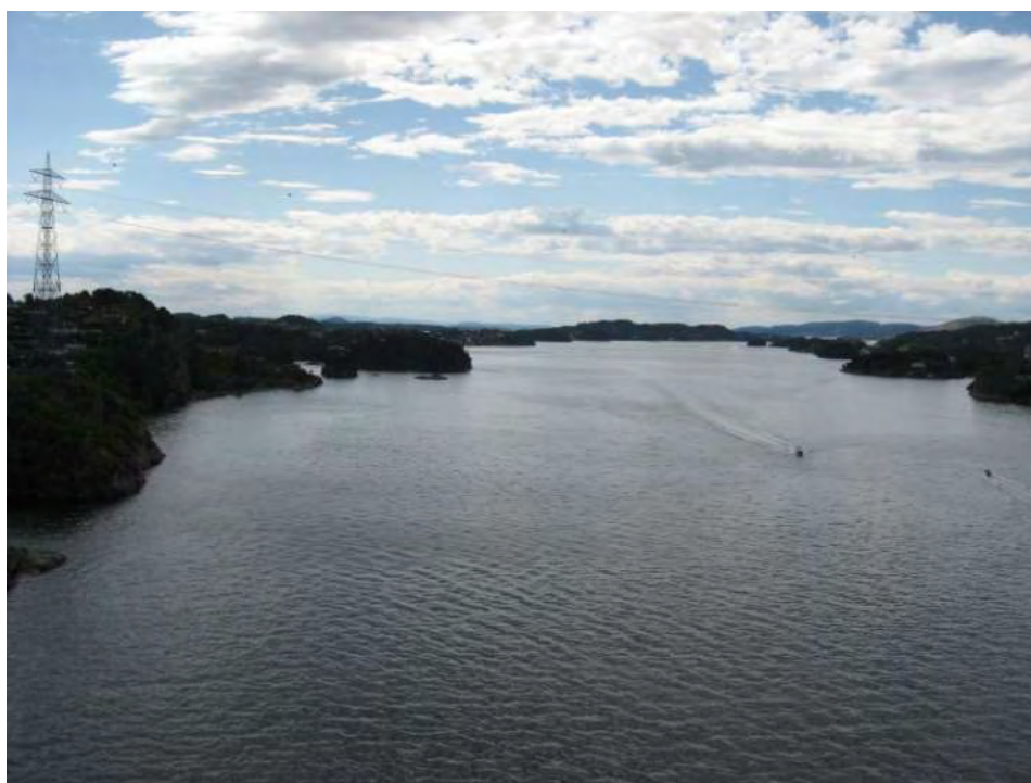
Figure 3: View southwards from the Sotra Bridge. During the test run discussed in the article, the wind was blowing from the south. The photo was taken on the bridge at the location of the white sonic anemometer (see Figure 3) (photo from Øiseth et al. 2013).
