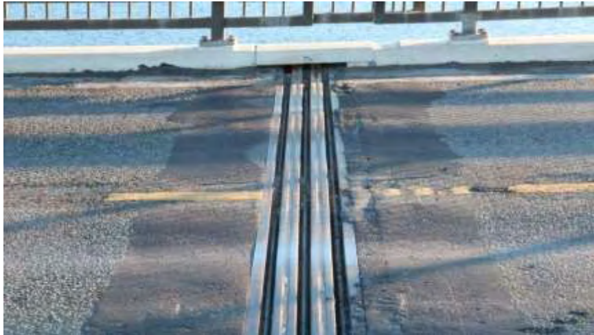
Figure 5 Road surface with upper viaduct joint (April 2013)
