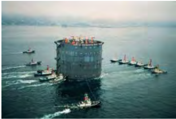
Photo 2 Towing of steel caisson to the site
