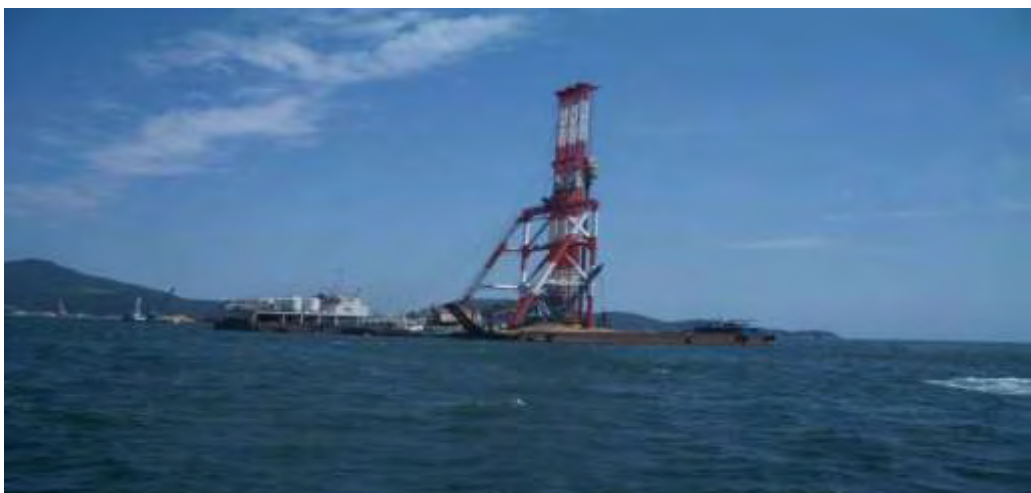
Fig. 3 Equipment for ground improvement in Busan
