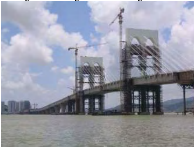
Fig. 6 Construction picture of the Saivan Bridge
