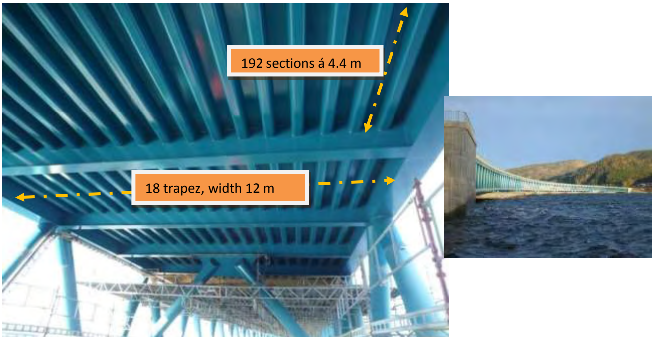
Photo no. 2 The orthotrop steel structure
