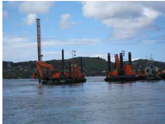
Fig.7. The drilling rig and the excavator.
