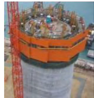
Figure 6: Lower Tower Construction
