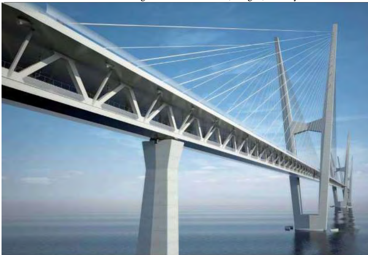
Figure 2 Proposed bridge solution for the Fehmarnbelt Fixed Link: Multi-span cable stayed bridge with two main spans of 724 m carrying two tracks of railway on the lower deck and four lanes of road traffic on the upper deck. Visualisation by Dissing+Weitling, courtesy of Femern Bælt A/S.
