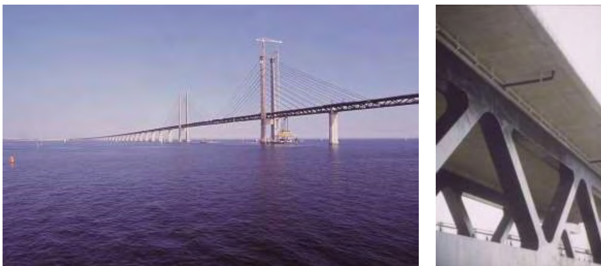
Figure 1 The Øresund Fixed Link between Denmark and Sweden, completed in 2000, carrying two tracks of railway on the lower deck and four lanes of road traffic on the upper deck. Courtesy of COWI A/S.
