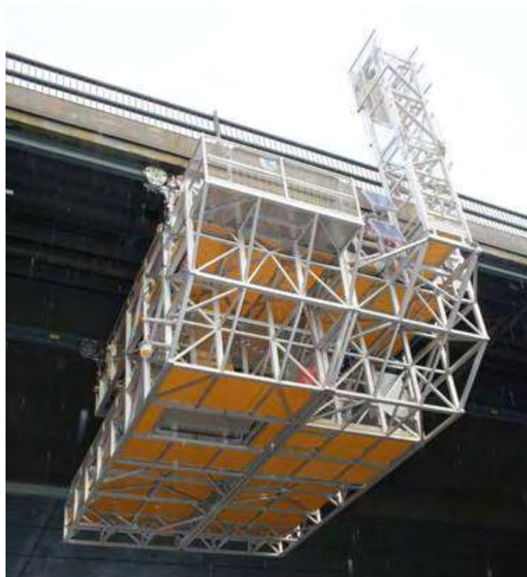
Figure 1 - Replacement Under Deck Gantry Solutions At Erskine Bridge
