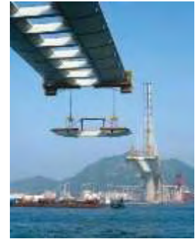
Figure 9: Two different methods were used in erecting the steel deck
