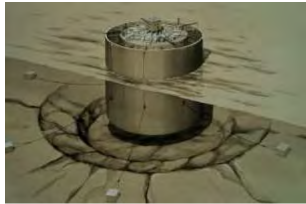
Fig.6 Installation of prefabricated steel caisson
