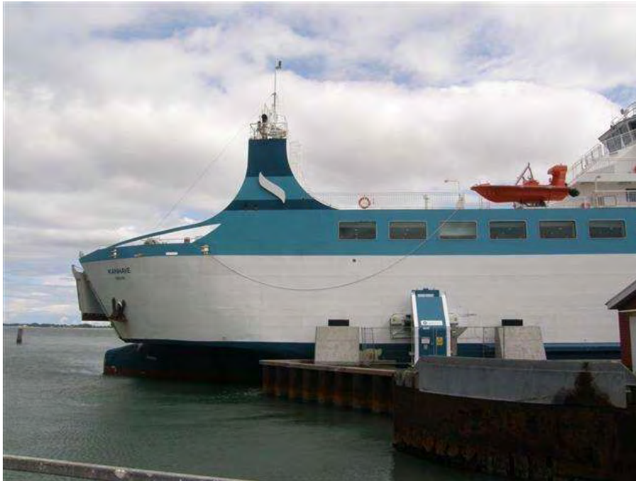
Figure 40: New Berth with Vessel Over-Hang
