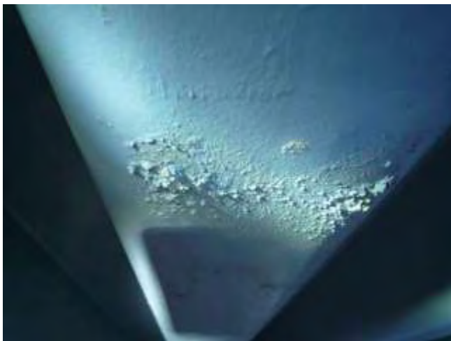
Photo no. 8 Penetration of corrosion products / blistering of the TSZ / coating (22 years)
