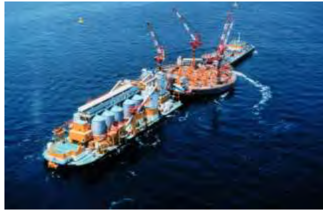
Photo 5 Casting of underwater concrete
