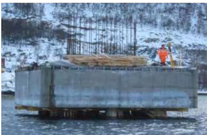
Figure 20 Left: Pile cap before installation of skirts. Right: Increased soil overburden.
