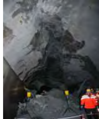
Figure 20 and 21: Technical requirements to prevent tunnel in operation from collapsing as in the Hanekleivtunnel, Norway 2006.
