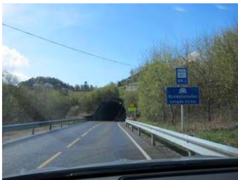
Fig2. The entrance to the Bjorøy tunnel.
