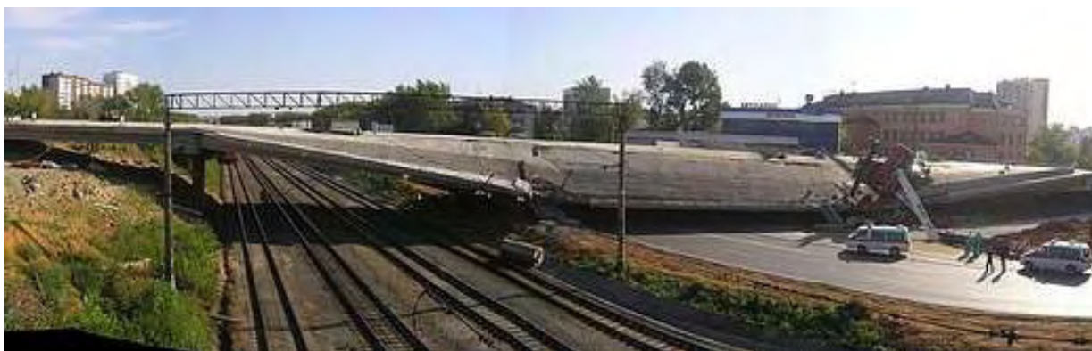
Figure 3. The destruction of the bridge in the city of Yekaterinburg
