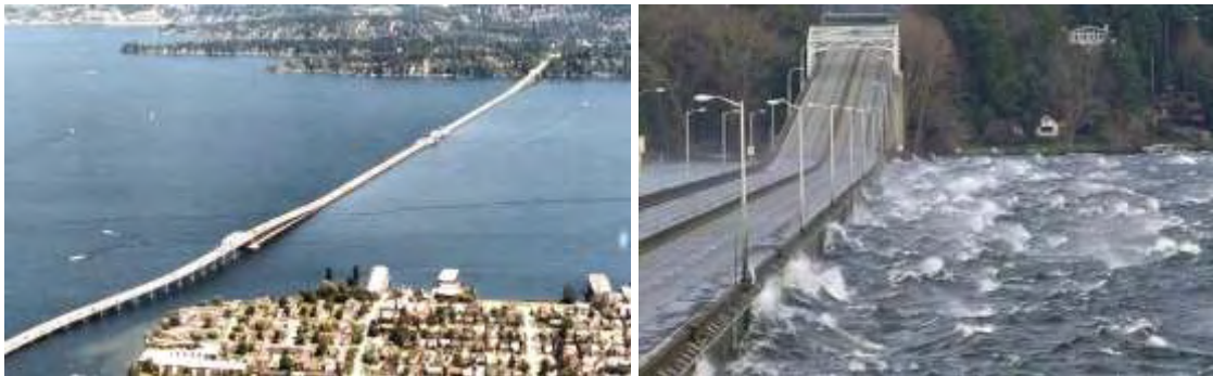
Figure 1 – Existing SR 520 Floating Bridge (looking to the east)
