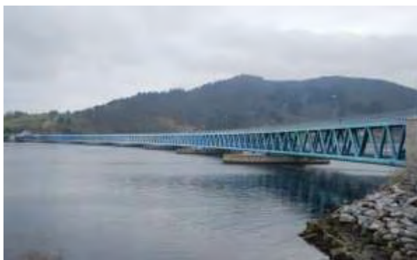
Figure 1. World first end anchored floating bridge – Bergsøysundet bridge – Norway.
