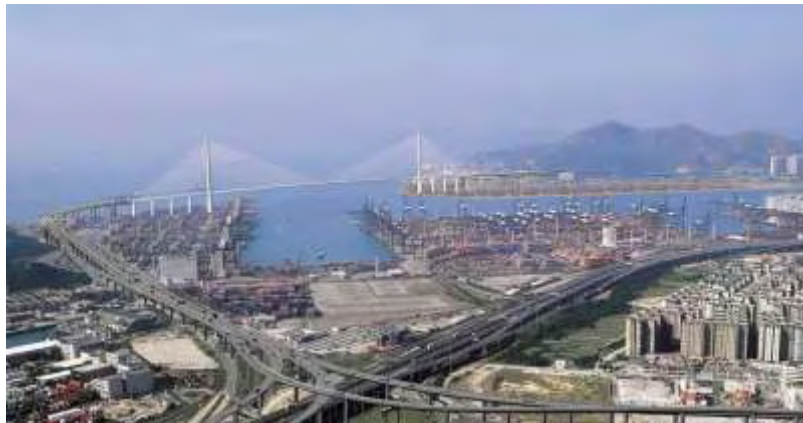
Figure 7 Artists view of the Stonecutters Bridge in Hong Kong
