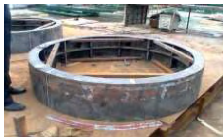
Fig.3 Preformed hole in the boxed bottom
