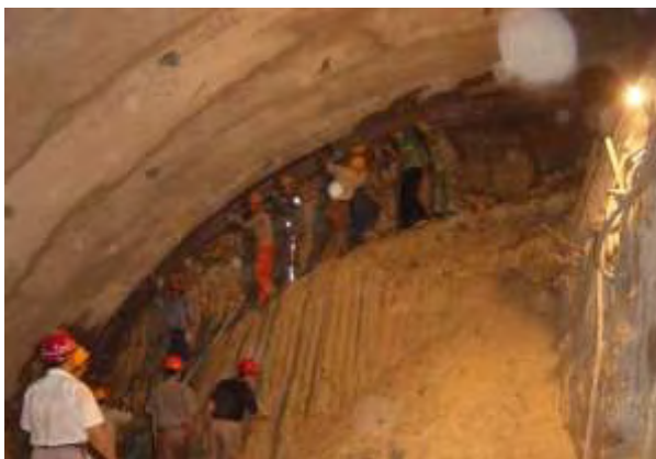
Fig. 10 Steel arch installation in roof and invert, and the soft ground condition.
