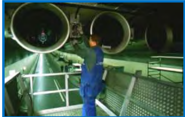
Figure 19: Maintenance works of tunnel ventilation
