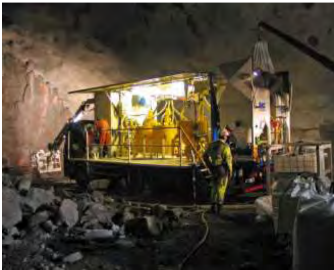
Figure 4. High pressure pre-grouting with modern grouting rig.
