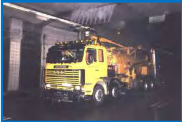
Figure 18: Tunnel washing by tunnel washing truck
