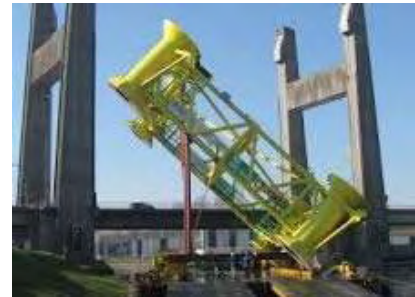
Figure 10 Pile Guiding Support Structure
