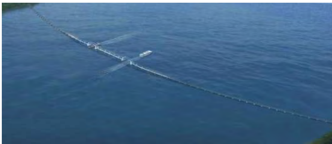
Figure 7 Floating bridge with two ship lane passages.
