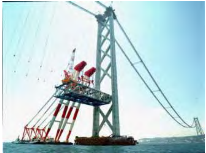
Photo 9 Large-block truss girder erection
