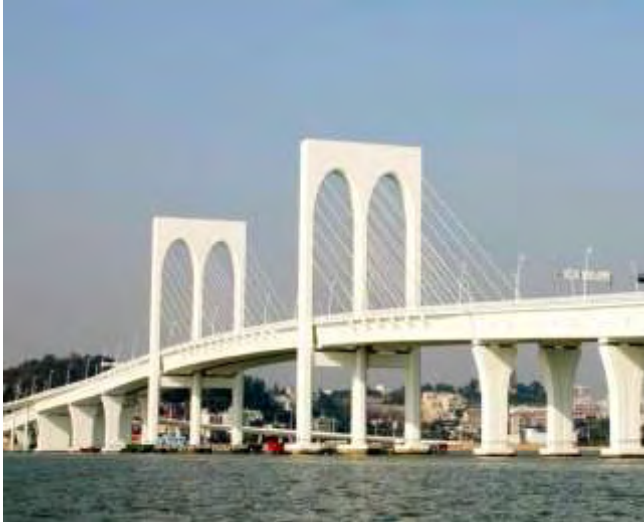
Fig.7 The General View of Saiwan Bridge
