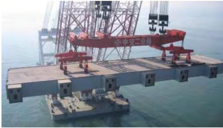
Fig.2 The four-point-hoisting and three-point-balance lifting tool
