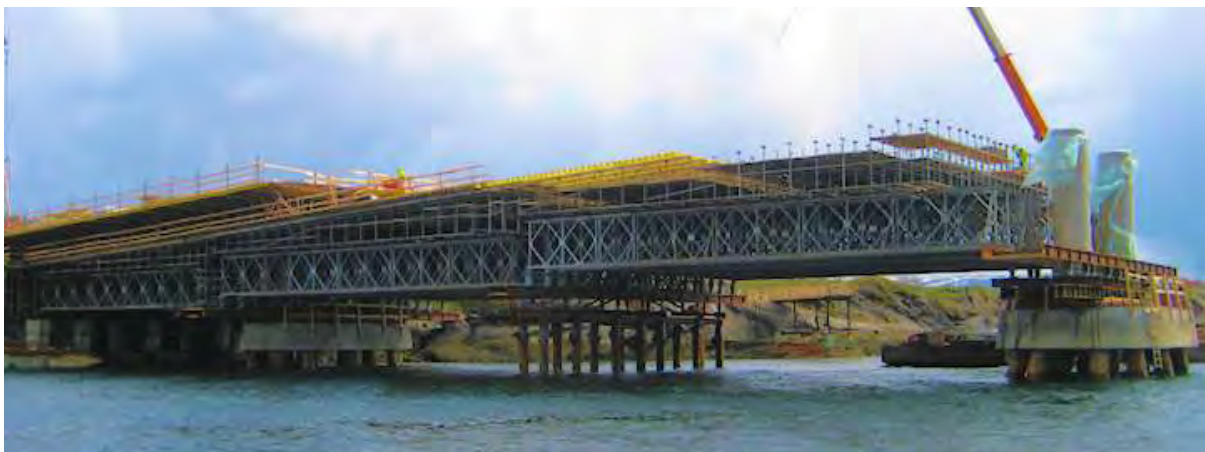
Fig. 8 Erection of Side Span
