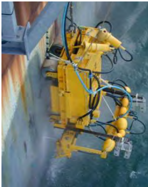
Figure 5 Cleaning machine for caisson wall
