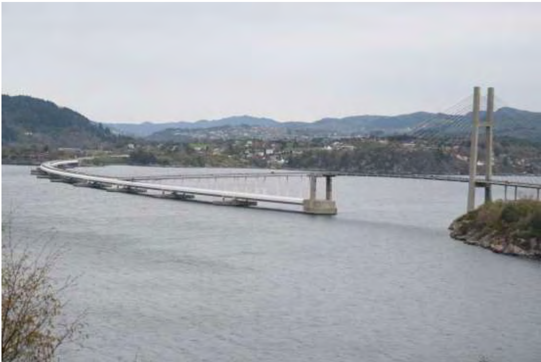
Figure 1 The Nordhordland Bridge
