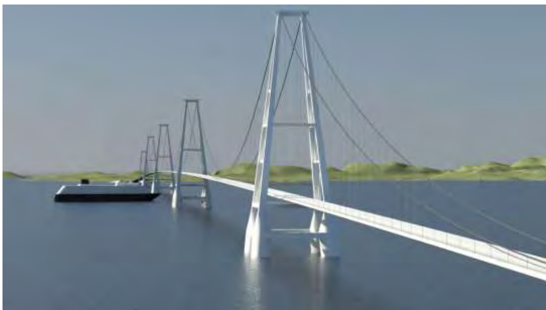
Figure 44: The 5 span suspension bridge crossing the Boknafjorden.
