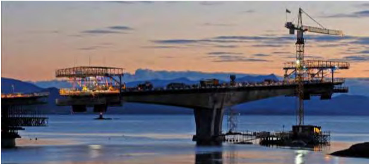
Fig. 6. Balanced Free Cantilevers Axis 4.
