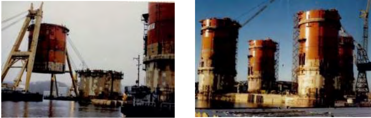
Fig. 4. Columns are lifted into position in Rosenberg Yard Stavanger.
