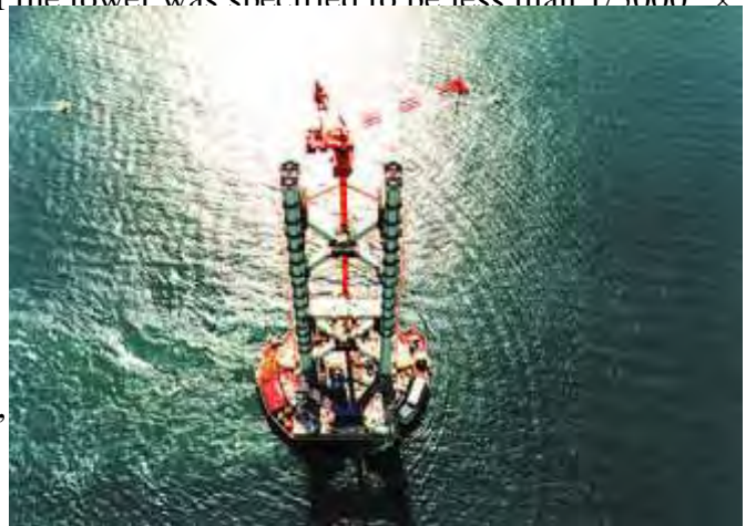
Photo 7 Erection of tower
