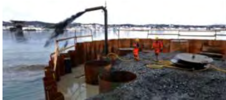
Fig. 3 Bored Piles Axis 2
