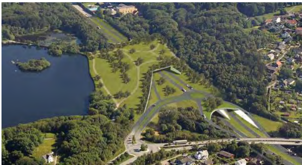
Figure 8 Southern portals to the Eiganes tunnel, and the Mosvannet Culvert (Land Bridge) north of the portal.
