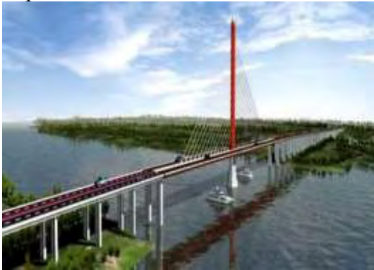
Fig.1 The Wusu Bridge panorama
