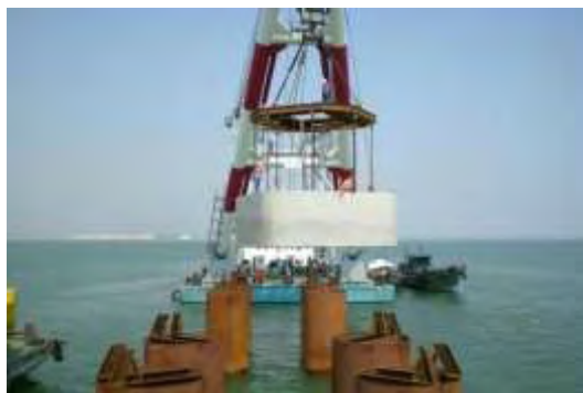
Fig.4 Installation of concrete cofferdam
