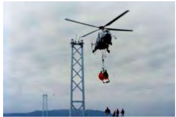
Photo 8 Pilot rope by a helicopter
