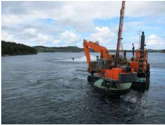
Fig.6. The excavating machine.
