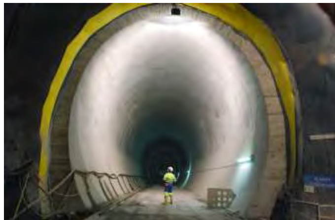
Figure 14: Inner lining of the Lötschberg Base Tunnel (Switzerland) [9].
