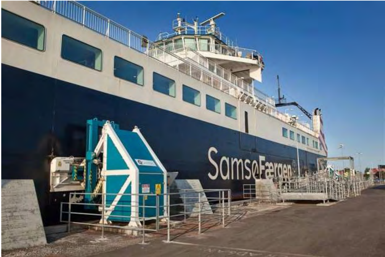
Figure 35: Typical Ferry Installation
