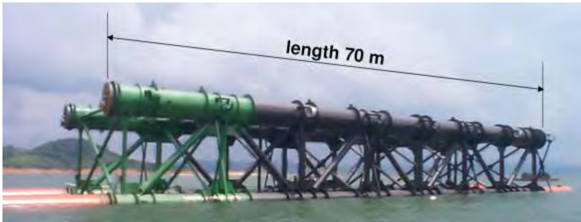
Figure 23 Jacket with buoyancy tanks 0.
