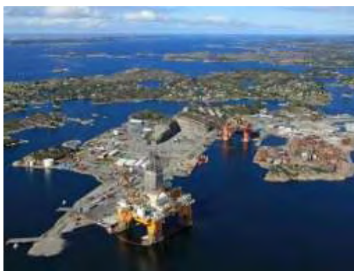
Fig. 8 Construction site, near Bergen
