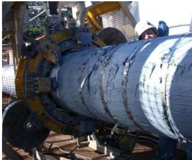
Figure 6 - Wrapping Main Cable Following Intrusive Inspection
