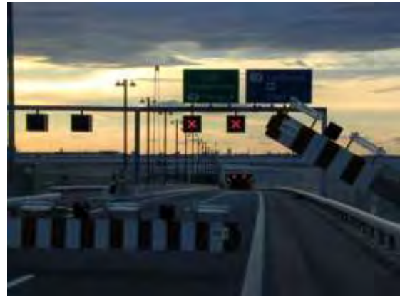
Figure 17: Preparation for cross over during night time.
