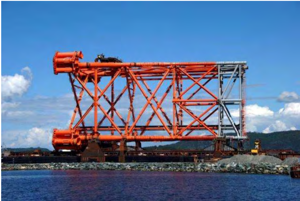
Fig. 10. Fabrication of a jacket on a yard.
