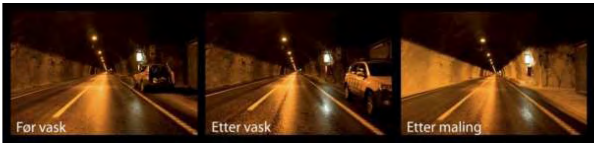
Figure 3: Arnanipa tunnel before washing, after washing of the whole tunnel, and after painting of walls
