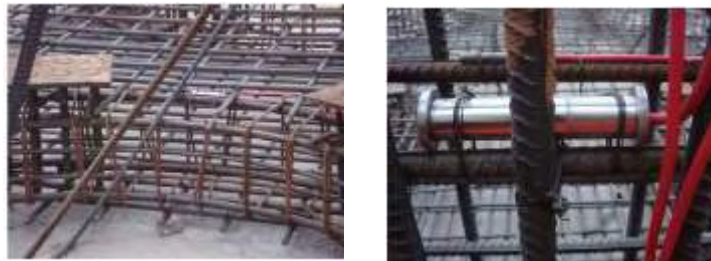
Fig.10 Sensors of boxes buried at the scene
