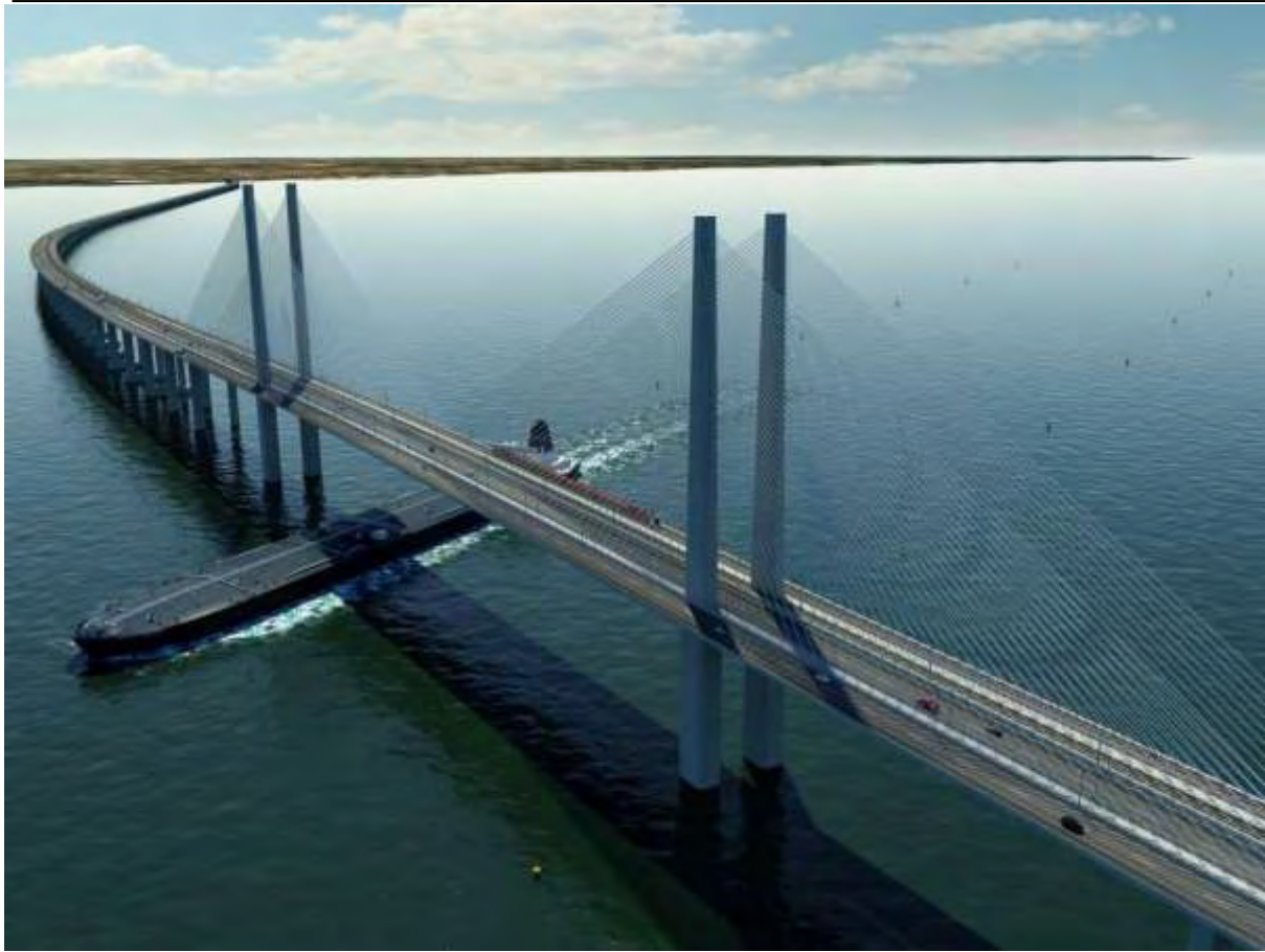
Figure 9 Puento Nigale, rendering showing the two main bridges across the navigation channel (rail bridge to the right). Courtesy of COWI A/S.
