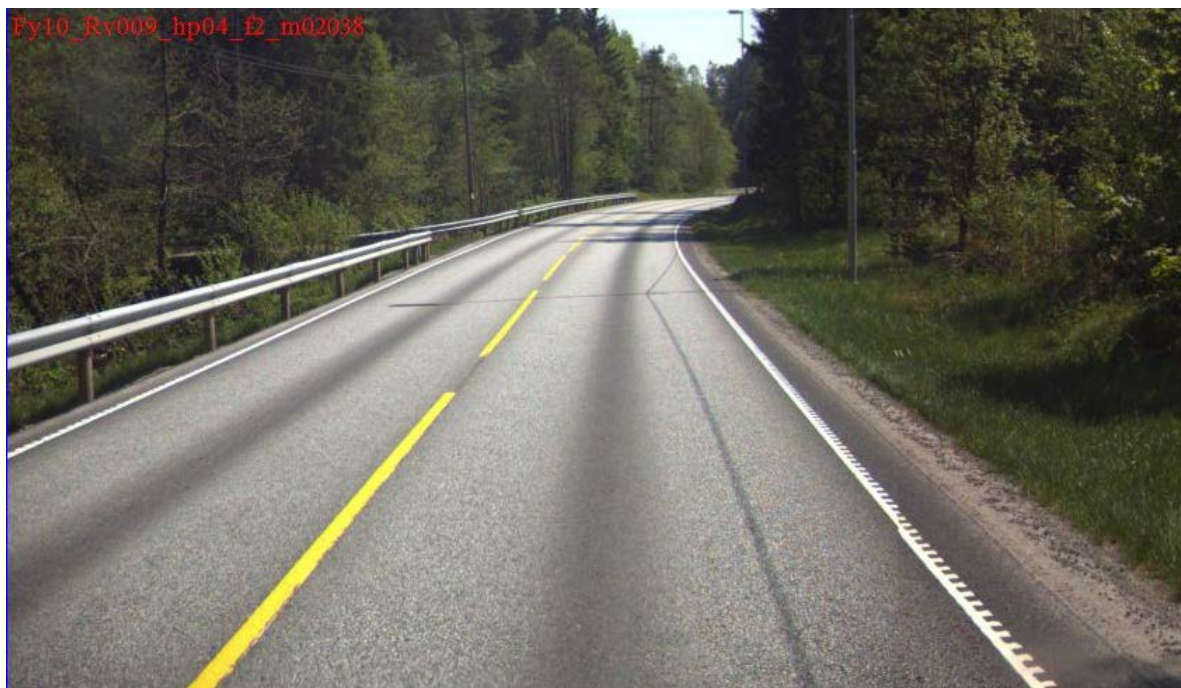
Figur 8. Rv 9, hp04/km 2,038_24.5.12. Ab16 Green Asphalt i felt 2.
