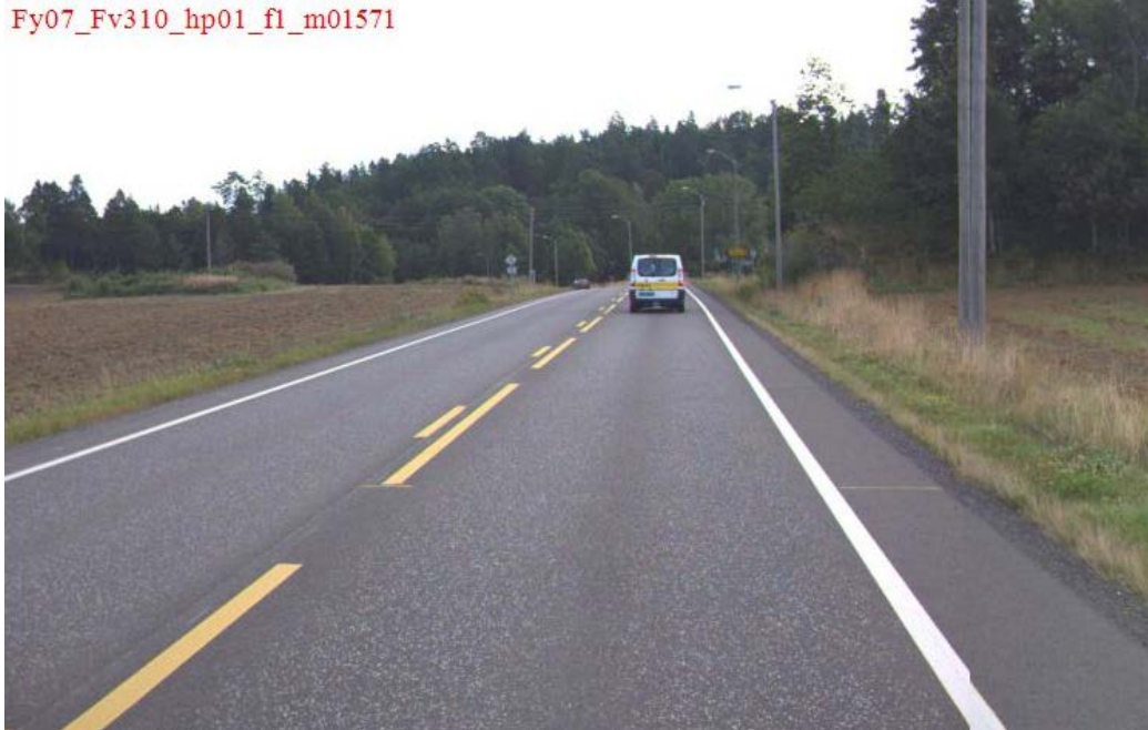
Figur 10. Fv. 310, hp01/km 1,571_21.8.12. Ab11 Cecabase 70/100 i felt 1.
