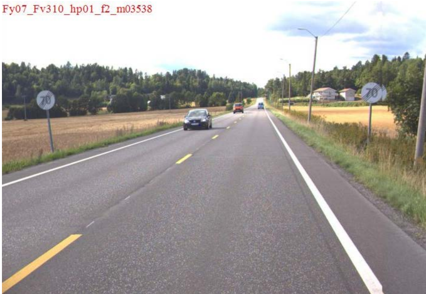
Figur 12. Fv. 310, hp01/km 3,538_21.8.12. Ab11 Cecabase 160/220 i felt 2
