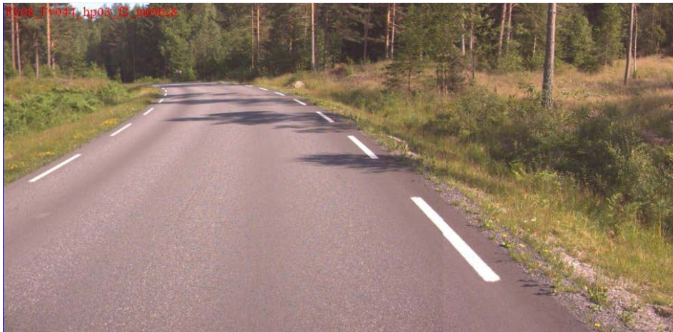
Figur 14. Fv. 44, hp03/km 9,628_21.8.12. Agb11 LMK skum i felt 2.
