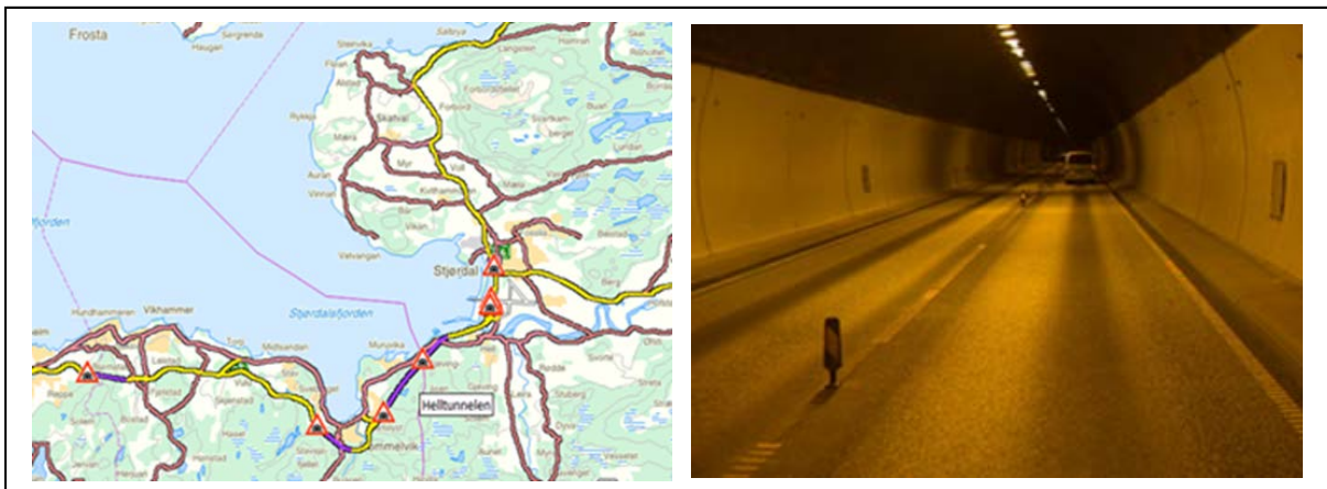
Figure 5: Hell tunnel, E6, Sør/Nord Trøndelag. Map and photography.
