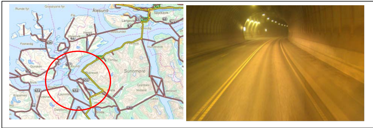
Figure 10: Eiksund tunnel, FV653, Møre og Romsdal. Map and photography.
