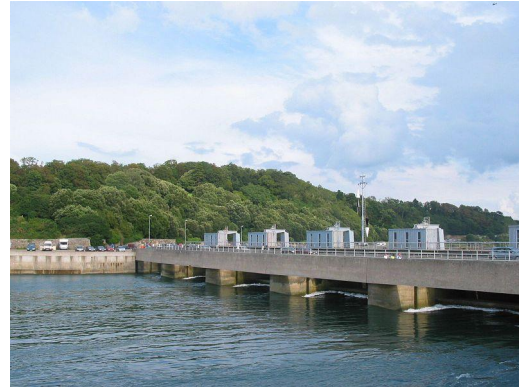
Picture of La Rance power station (Wikipedia)
