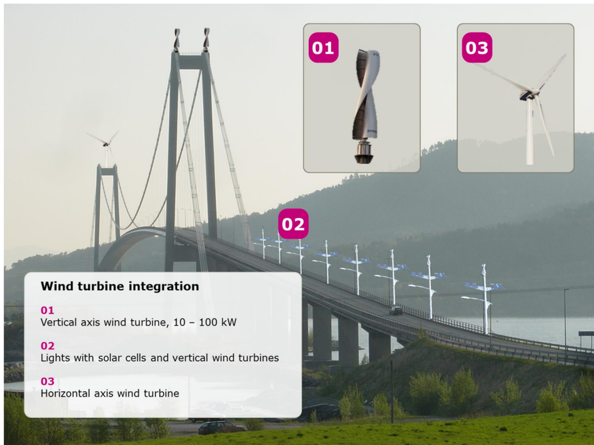
Figure 4-1 Wind turbine integration on a suspension bridge
