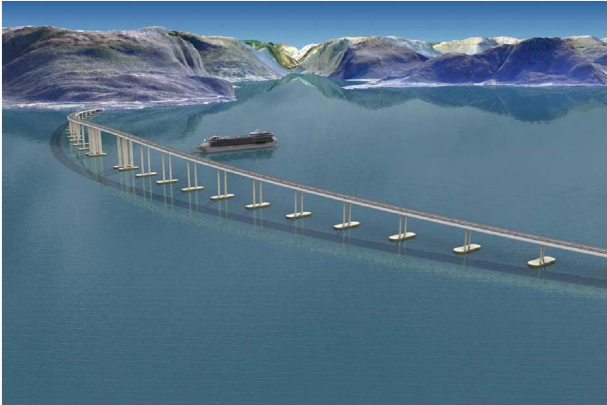
Figure 2-3 Floating (pontoon) bridge (SVV)
