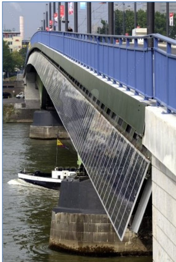
Kennedy Bridge (Bonne, Germany). Walkway bridge completed 2011 392 panels installed (Solarworld)
